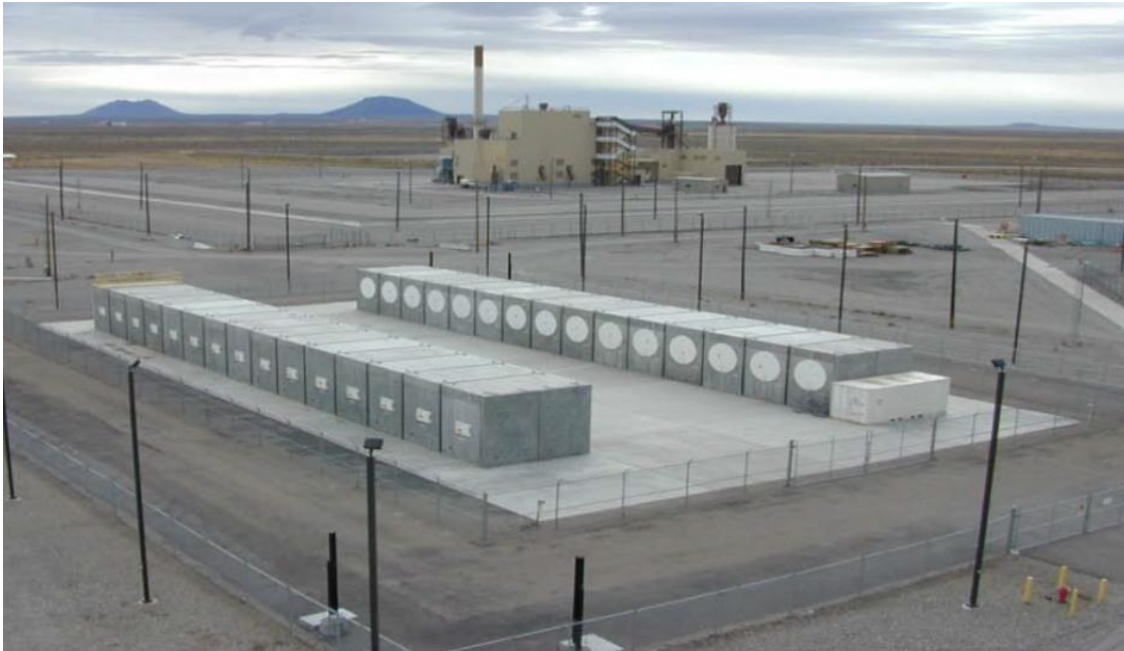
Figure 2-9. NUHOMS Dry Storage Casks Emplaced in Concrete Horizontal Storage Modules at the Idaho National Laboratory Independent Spent Fuel Storage Installation (Photo courtesy of Idaho National Laboratory)
