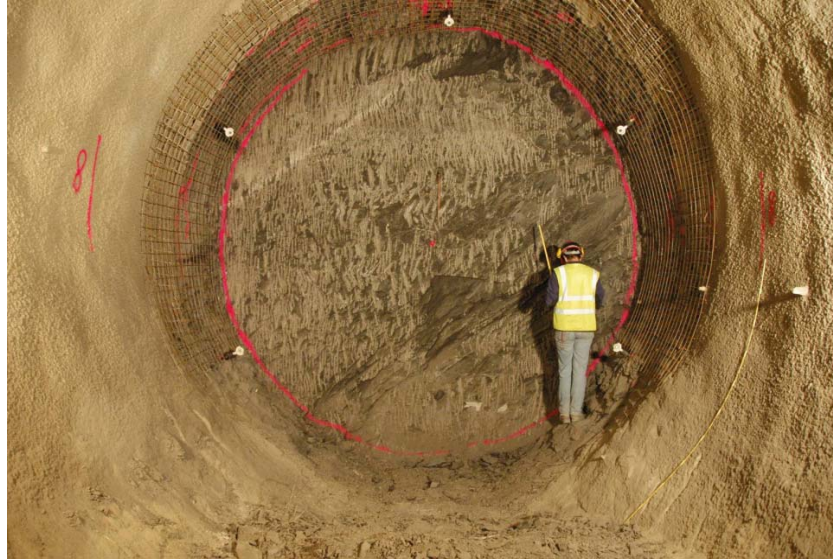
Figure 4-5. View of FE tunnel face from the FE niche showing beddings dipping 45° (Vieter, 2012).
