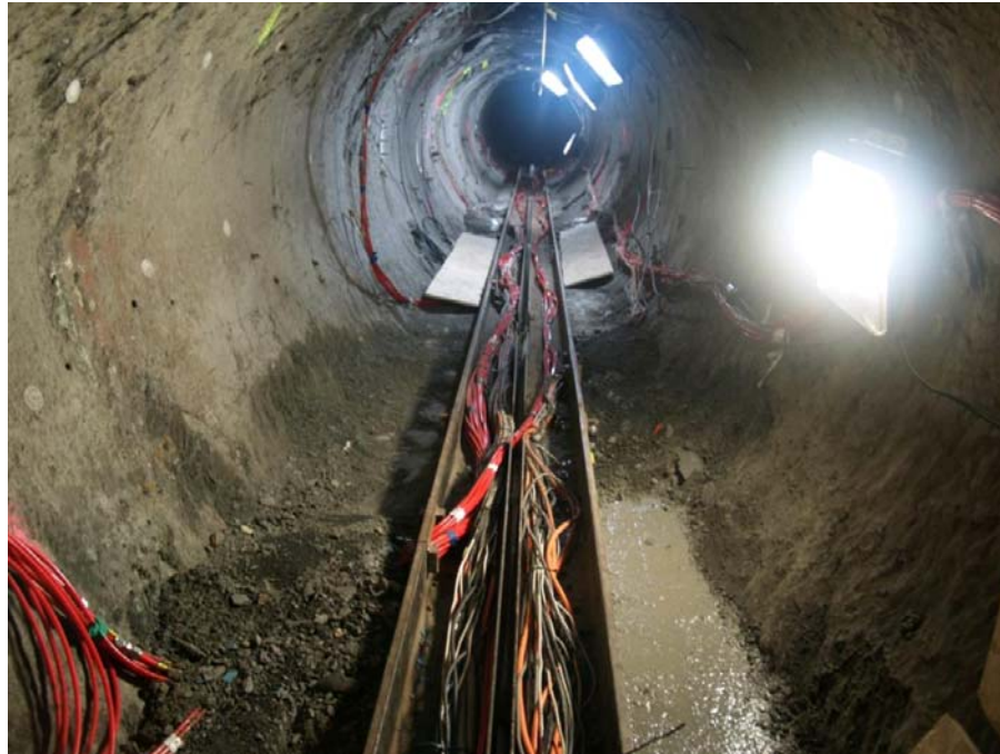
Figure 3-7. HE-E Heater Test at Mont Terri URL: Photo of micro-tunnel before buffer emplacement (from Gaus et al., 2012)
