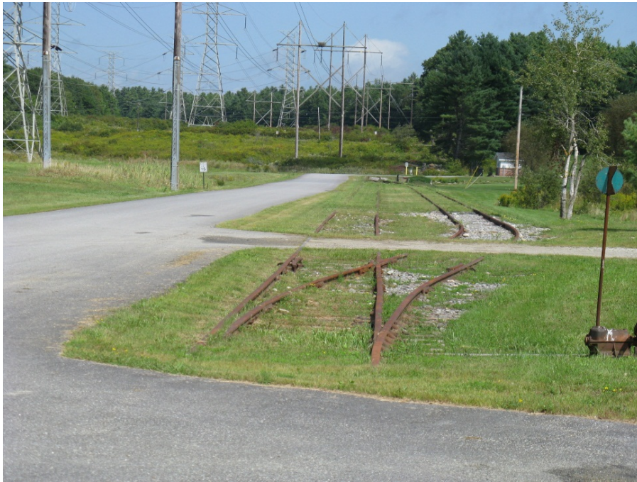
Figure 3-3. Paved-over Railroad Tracks at the Maine Yankee Site
