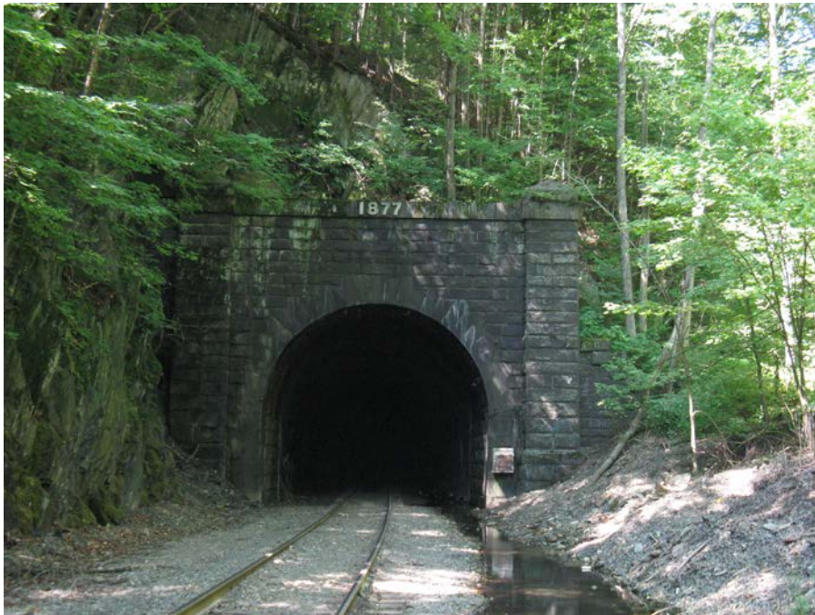
Figure 4-11. East Portal of the Hoosac Tunnel
