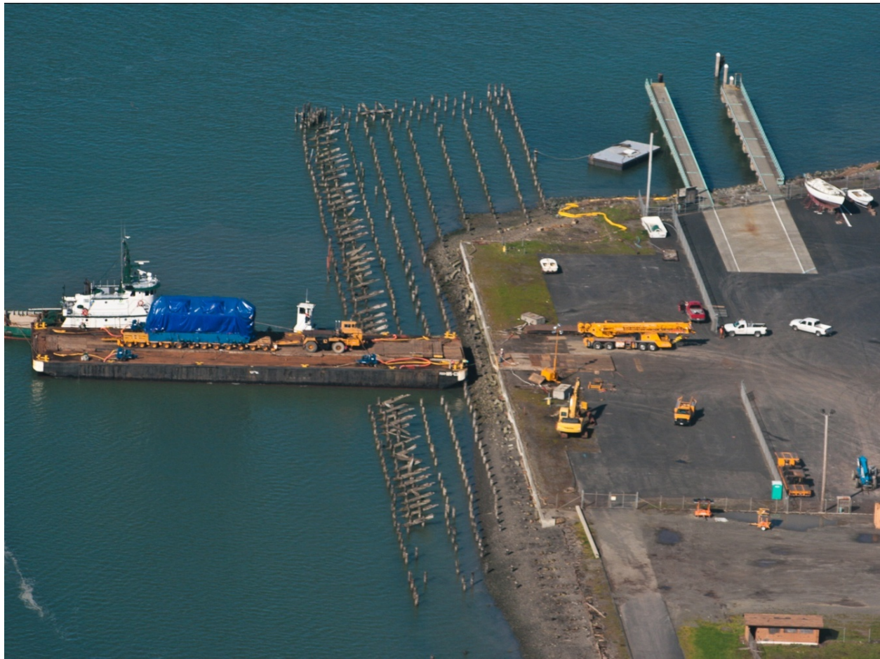
Photo courtesy of Bragg Crane & Rigging Co.
