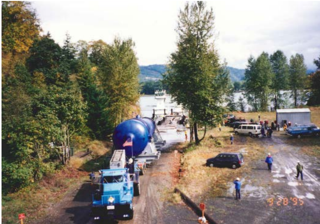
Photo courtesy of Portland General Electric Company
