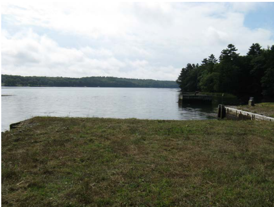
Figure 3-4. Barge Dock at the Maine Yankee Site
