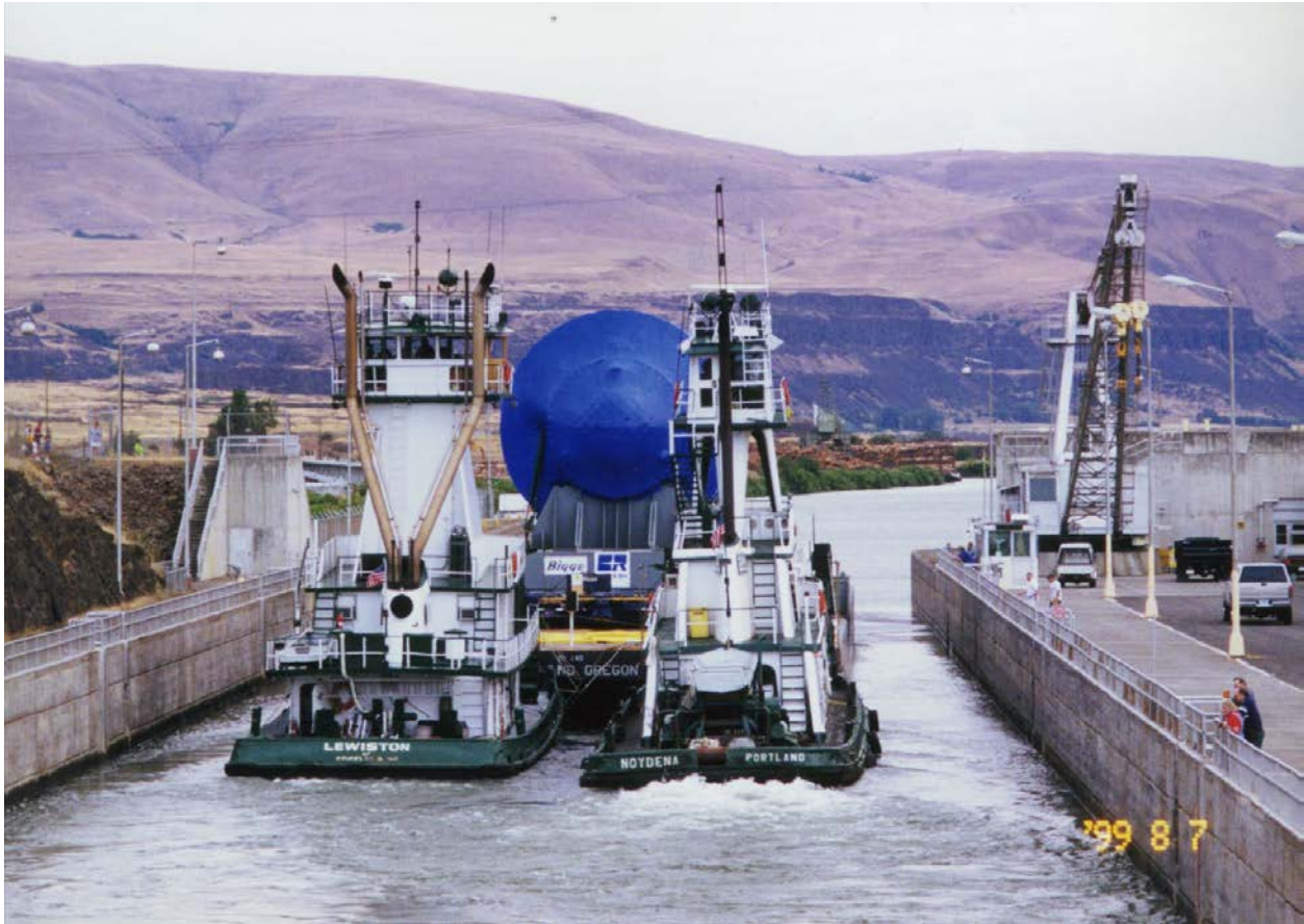
Photo courtesy of Portland General Electric Company
