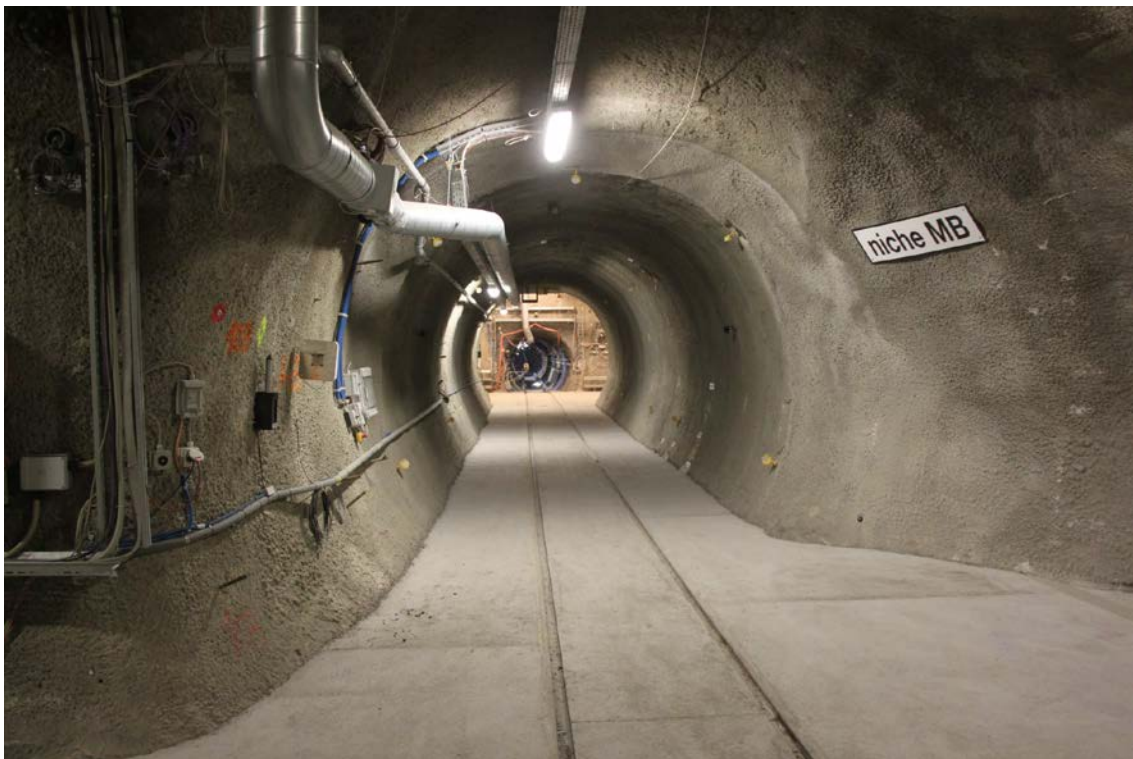
Figure 3.1-7 View from the FE gallery into the heater tunnel during final installation (Bossart 2014a).
