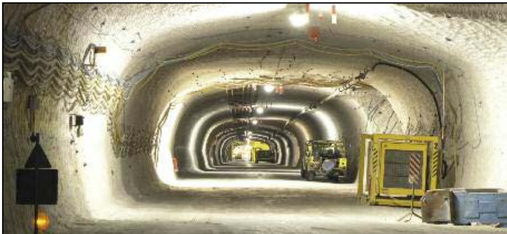
Figure 4.2-1 View of one of the underground tunnels at Gorleben at the 840 m level (BMW 2008).
