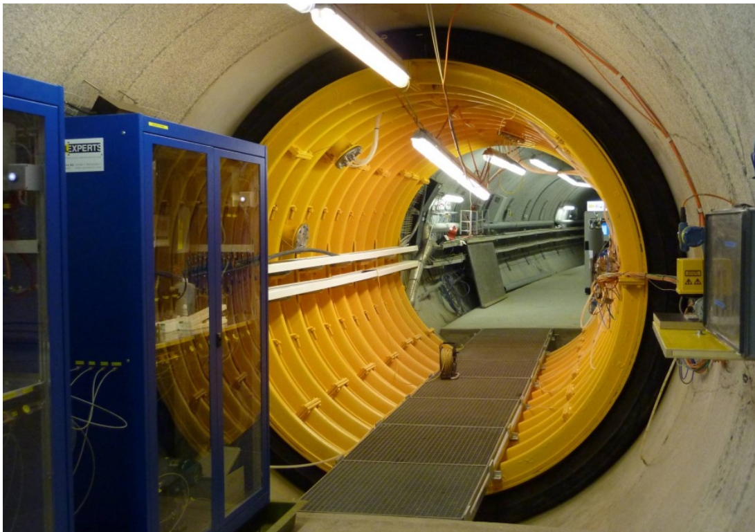
Figure 3.3-3 CFM field test bed at Grimsel Test Site: Tunnel packer system used to isolate the shear zone ( http://www.grimsel.com/gts-phase-vi/cfm-section/cfm-site-preparation ). Small disks with tubing issuing from them (inside yellow packer) are “surface packers” that seal the tunnel wall and collect water from inflow points. Tunnel diameter is 3.5 meters.
