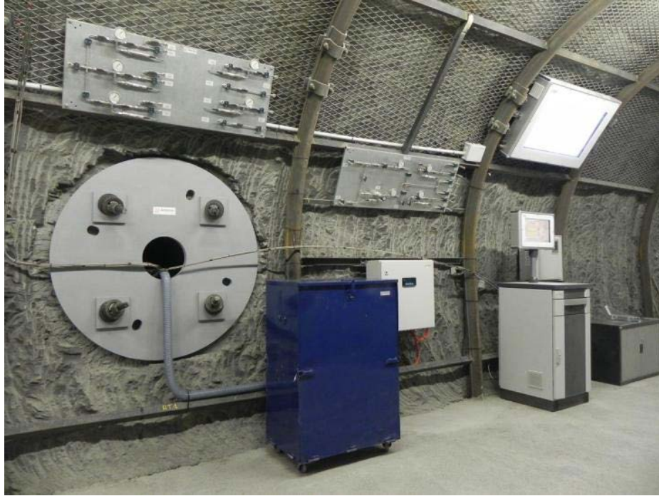
Figure 3.2-3 SEALEX Experiment at the Tournemire URL: View of mini-tunnel from gallery after seal emplacement (Barnichon 2011).
