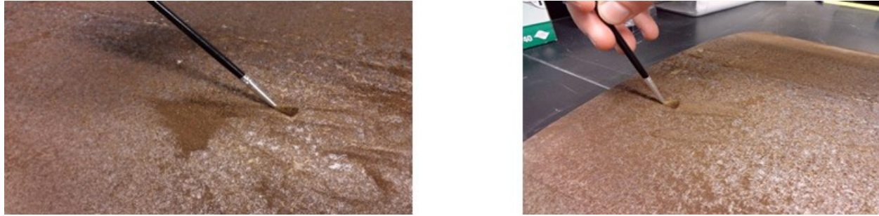
Figure 45. Image of mock-up canister plate after 8-month exposure time to 80°C, 35 % RH showing the surface of the plate to be completely dry. The images show the removal of the loose corrosion products with a small brush.
