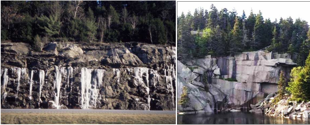
Figure 4-7. Examples of horizontal fractures in crystalline rocks of southern Maine. Left: Groundwater flow (icicles) from a horizontal fracture exposed in a roadcut near Falmouth, Maine (MGS 2012). Right: horizontal fractures exposed in a quarry face in the Vinalhaven Pluton, Hurricane Island, Maine (Lemmond 2016).
