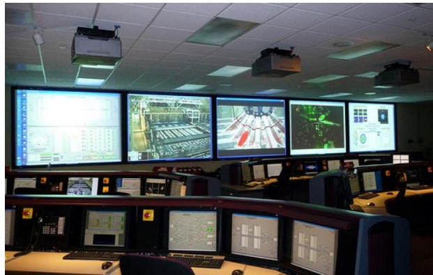
Figure 5-10 Representative Facility MCR Operator Console, PCS Displays & Overhead Status, Process, and Annunciator Displays
