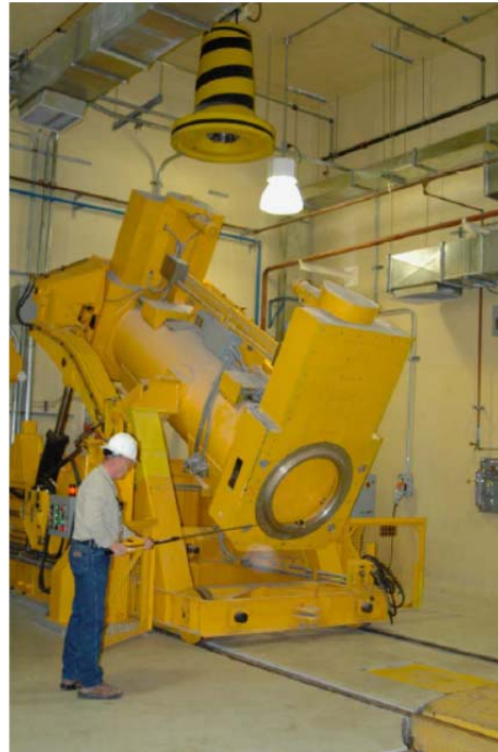
Figure 5-23 The Facility Cask Containing The Waste Canister Is Rotated To A Horizontal Position Prior To Transfer Onto The Waste Shaft Hoist Conveyance
