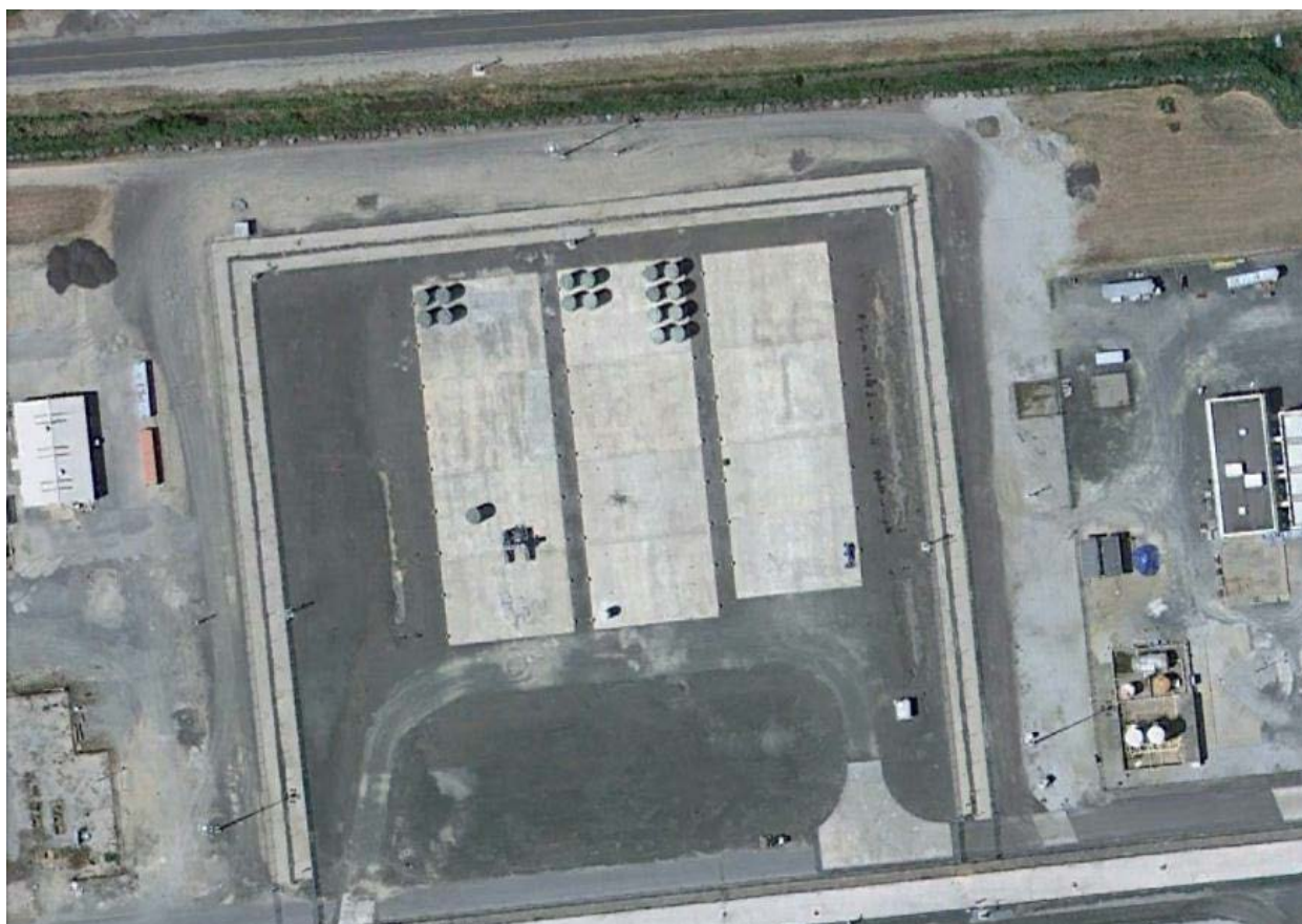
Figure 1-1. Aerial View of Hope Creek Nuclear Generating Station ISFSI, Showing Arrays of Vertical Storage Modules (Google 2011)
