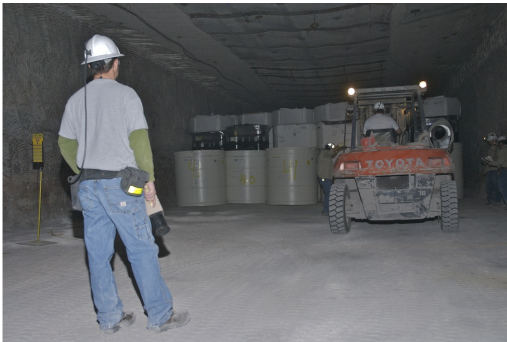
Figure B-9. CH waste being disposed in a disposal room at WIPP
