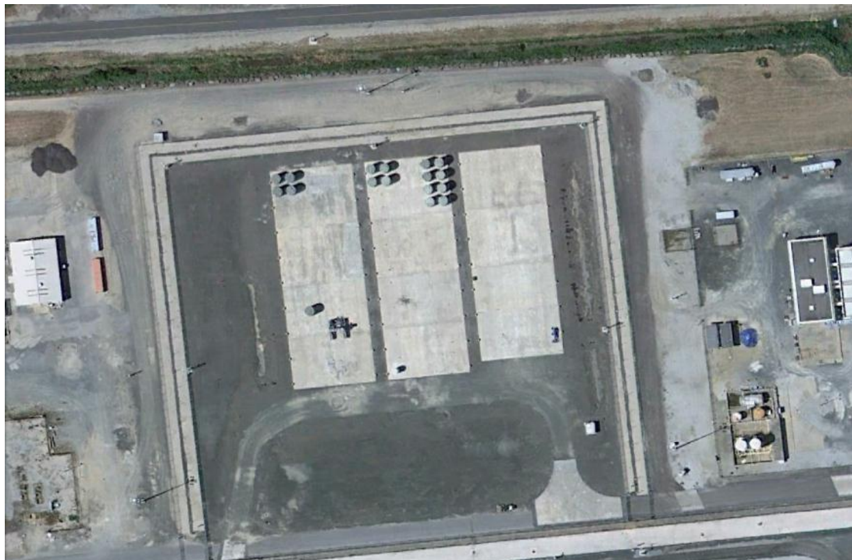
Figure 1-1. Aerial View of Hope Creek Nuclear Generating Station ISFSI, Showing Arrays of Vertical Storage Modules (Google Earth 2011)
