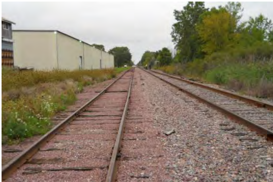
Figure B-26. Wall Street Siding in Bellevue, Wisconsin (2014)
