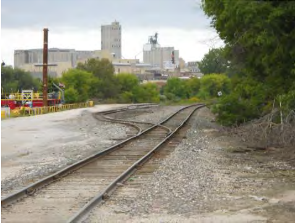
Figure B-37. Red Arrow Siding (2014)
