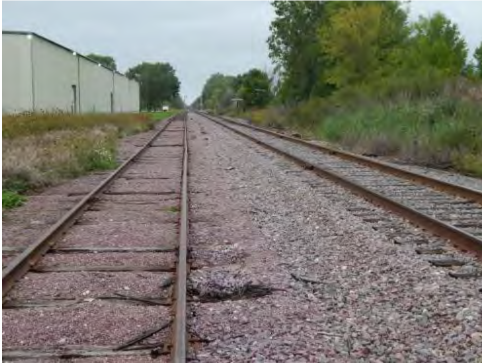
Figure 2-213. Potential Bellevue Transload Location (Looking North) (2014)
