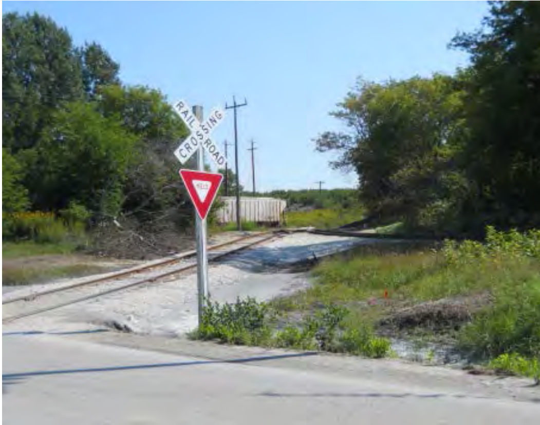
Figure B-32. Switch to Carmeuse Lime Plant and the Country Visions Cooperative Fertilizer Plant Sidings at MP 83.2 (2014)
