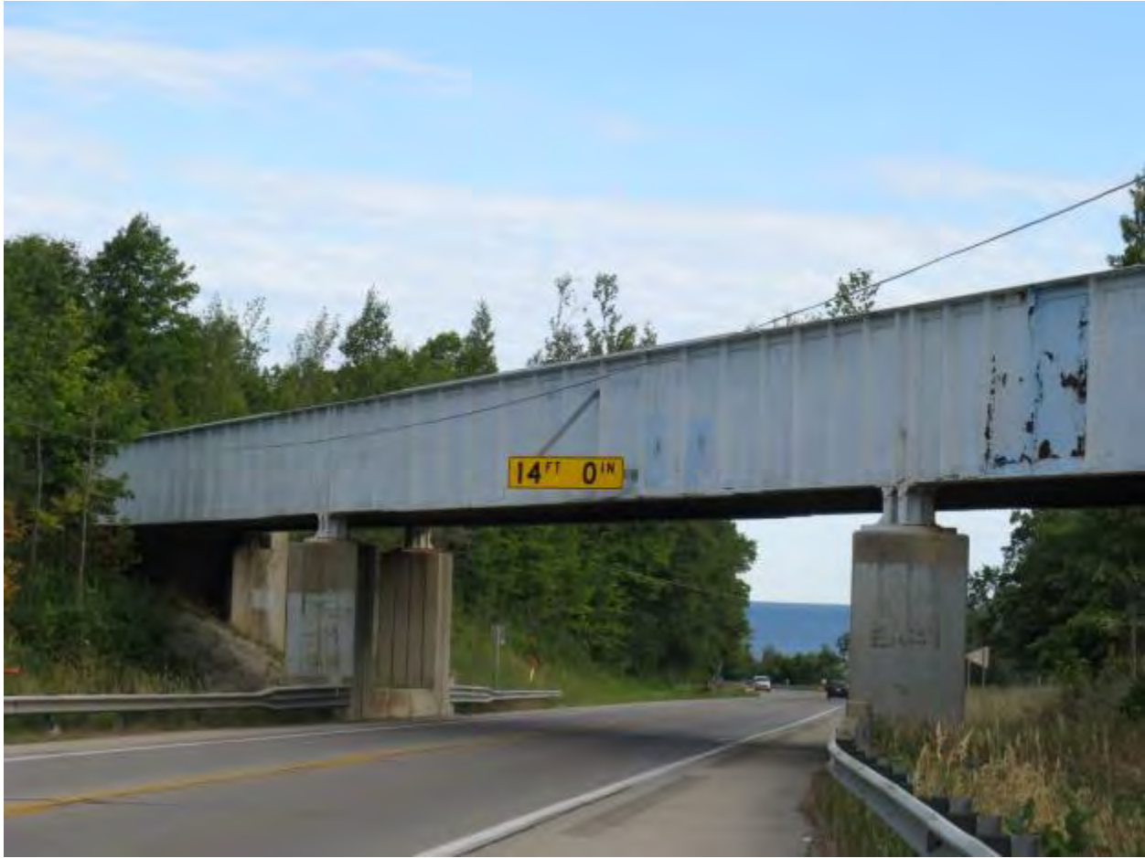
Figure 2-73. Low Overhead Clearance Abandoned Railroad Bridge on U.S. 31 (2013)
