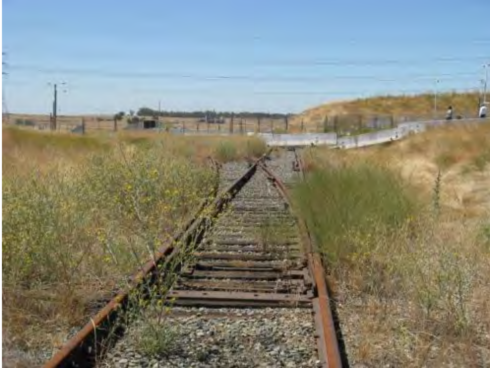
Figure 2-89. Junction of the On-site Track Spur Running Adjacent to the Independent Spent Fuel Storage Installation (Right) and the Longer Track Running into the Rancho Seco Site (Left) (2013)
