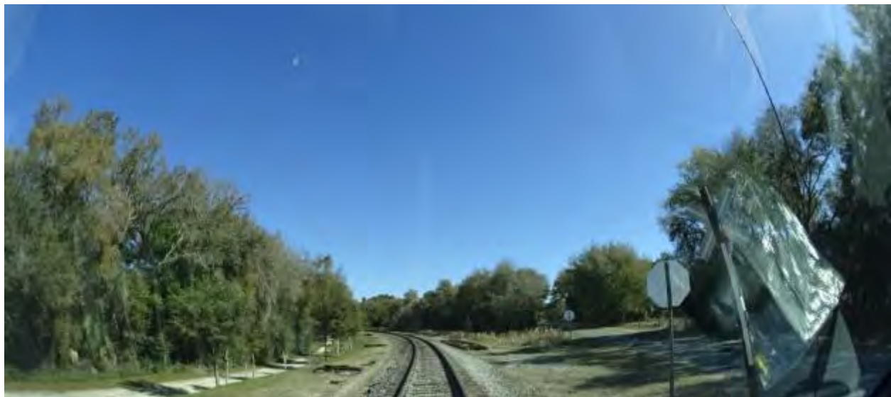
Figure 2-166. Florida Northern Railroad near Dunnellon, Florida (2015)
