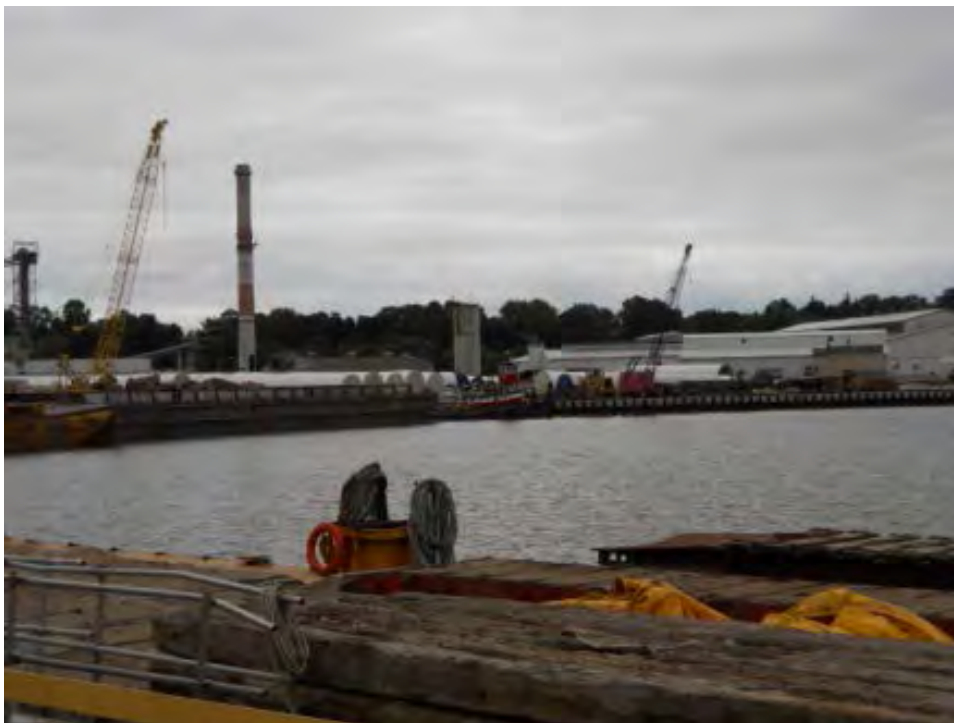
Figure B-38. Barge Slip Adjacent to Red Arrow Siding (2014)
