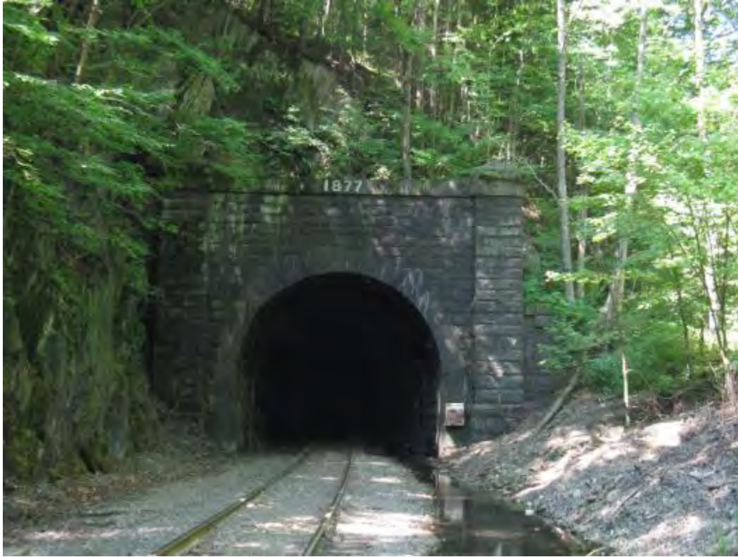
Figure 2-26. East Portal of the Hoosac Tunnel (2012)
