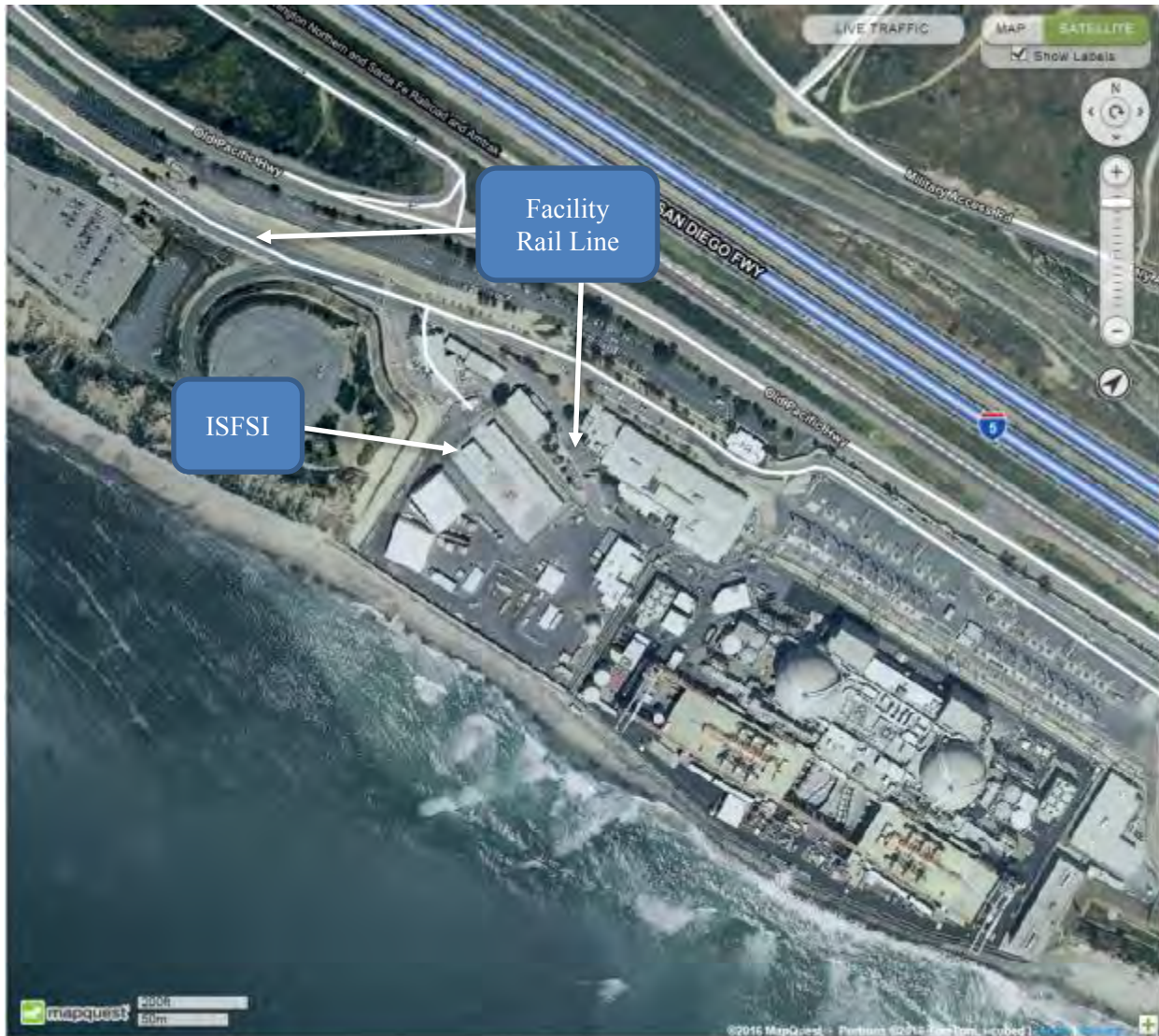
Figure B-50. San Onofre Site ISFSI and Facility Rail Line (MapQuest 2016)
