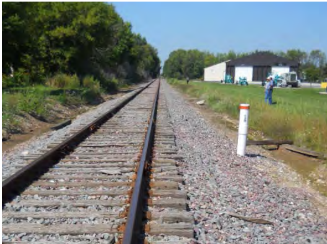
Figure B-33. Manitowoc County Highway Maintenance Facility at MP 82.14 (2014)
