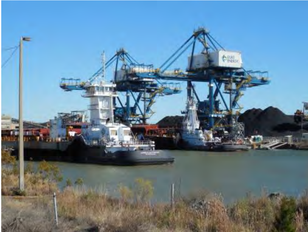
Figure 2-161. Current Barge Area Used for Unloading Coal Barges (2015)
