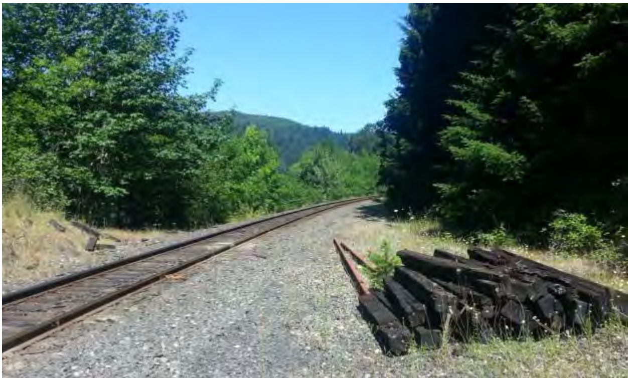
Figure 2-106. Location of Former Junction of Portland and Western Railroad and Trojan Rail Spur (2013)
