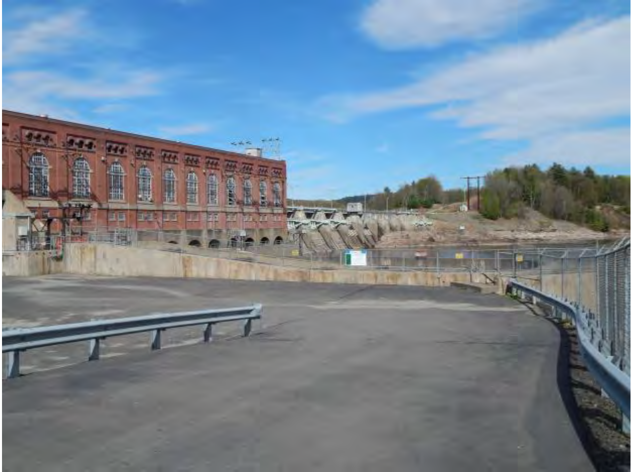
Figure 2-302. Vernon Dam and Hydroelectric Station (2016)
