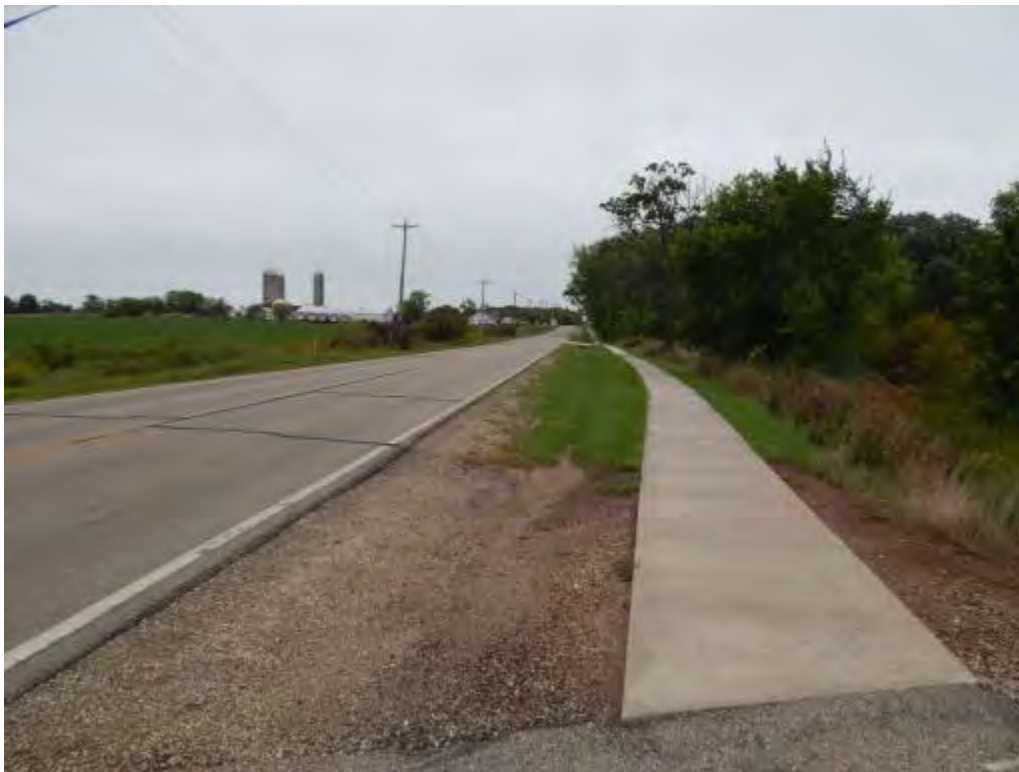
Figure 2-224. Potential Denmark Transload Location (Looking East) (2014)
