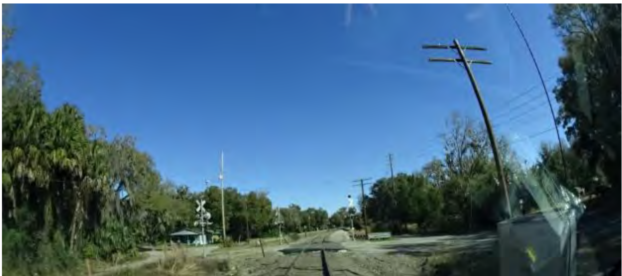
Figure 2-168. Florida Northern Railroad Grade Crossing (2015)
