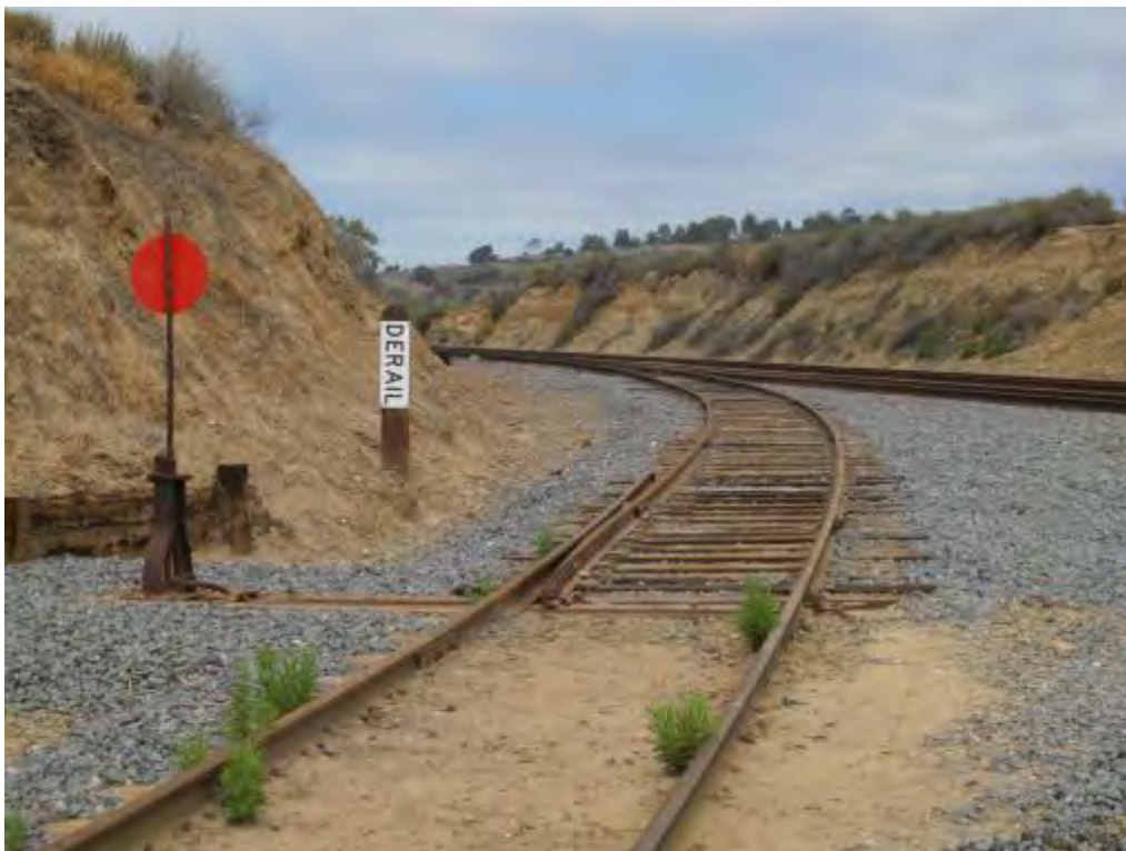
Figure 2-280. Junction of Onsite Rail Spur with Mainline at San Onofre Site (2015)
