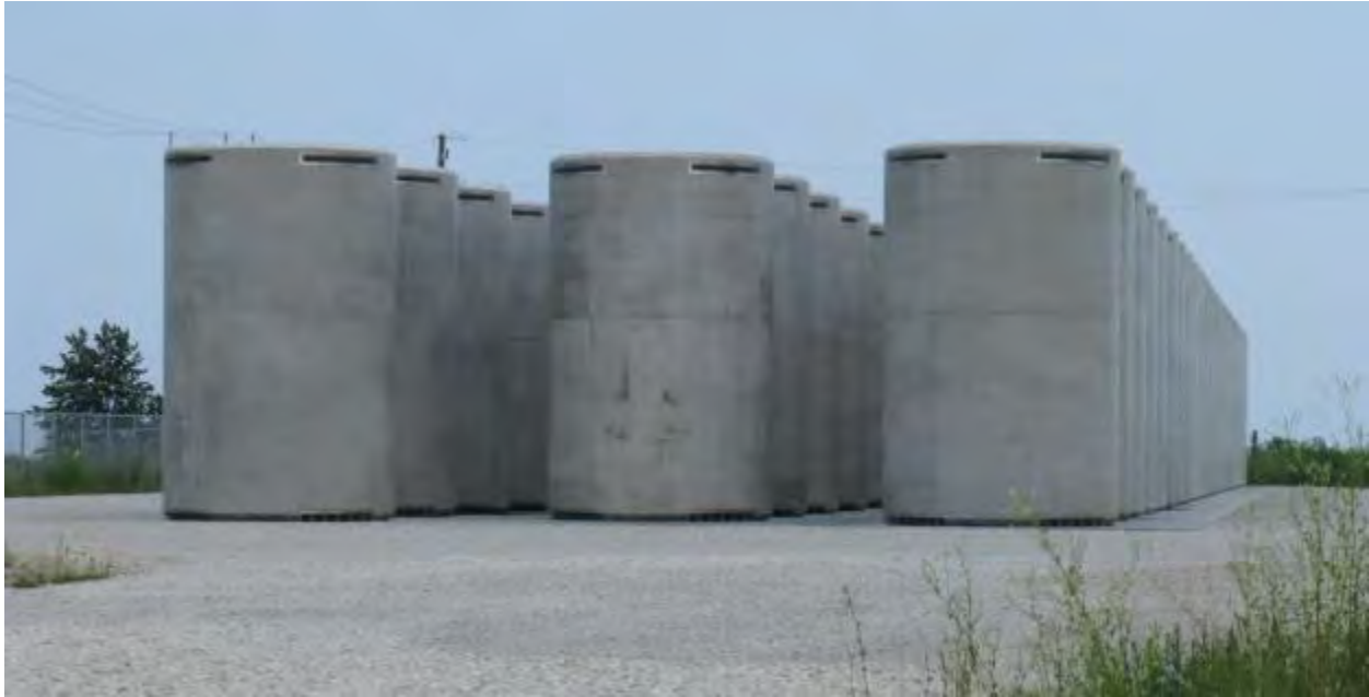
Figure 2-137. Vertical Concrete Storage Casks Staged at Zion (2013)
