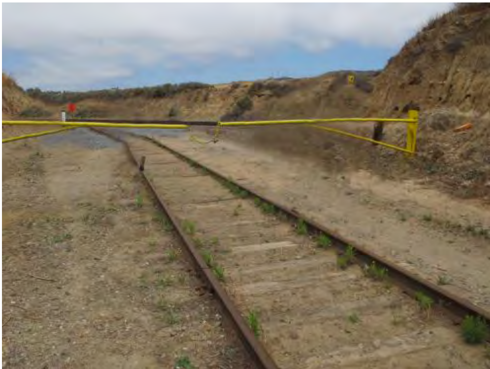
Figure B-58. Locked Facility Gate (2015)
