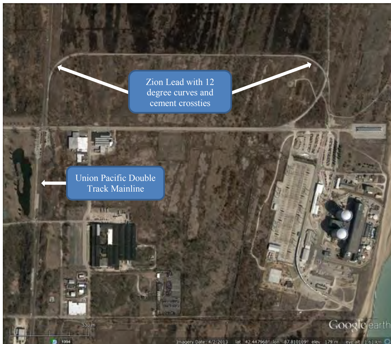
Figure B-22. Satellite View of the Zion Lead and the Union Pacific Double Track Mainline (Google 2015)
