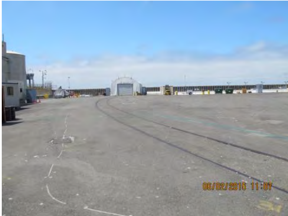
Figure 2-277. Onsite Rail System near Independent Spent Fuel Storage Installation at San Onofre Site (Looking Southwest) (2015)
