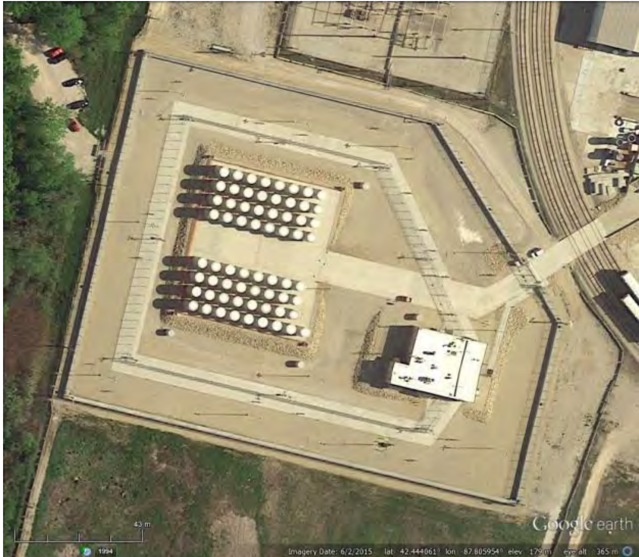
Figure 2-136. Aerial View of Zion Independent Spent Fuel Storage Installation (Google 2015)
