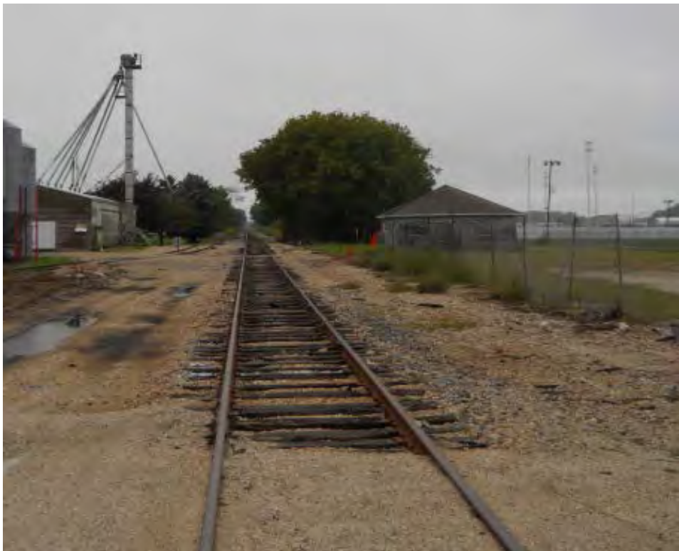
Figure B-42. Main Track at Luxemburg (2014)
