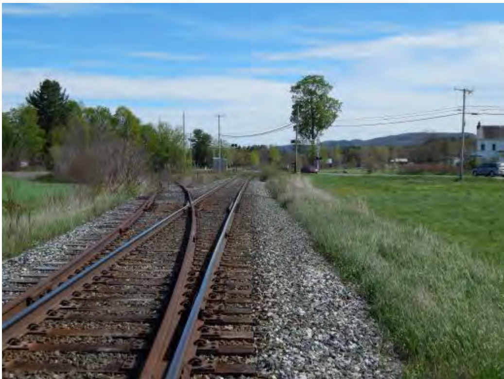
Figure 2-314. Junction of Vermont Yankee Rail Spur (Left) and New England Central Railroad Mainline (Right) Looking South (2016)
