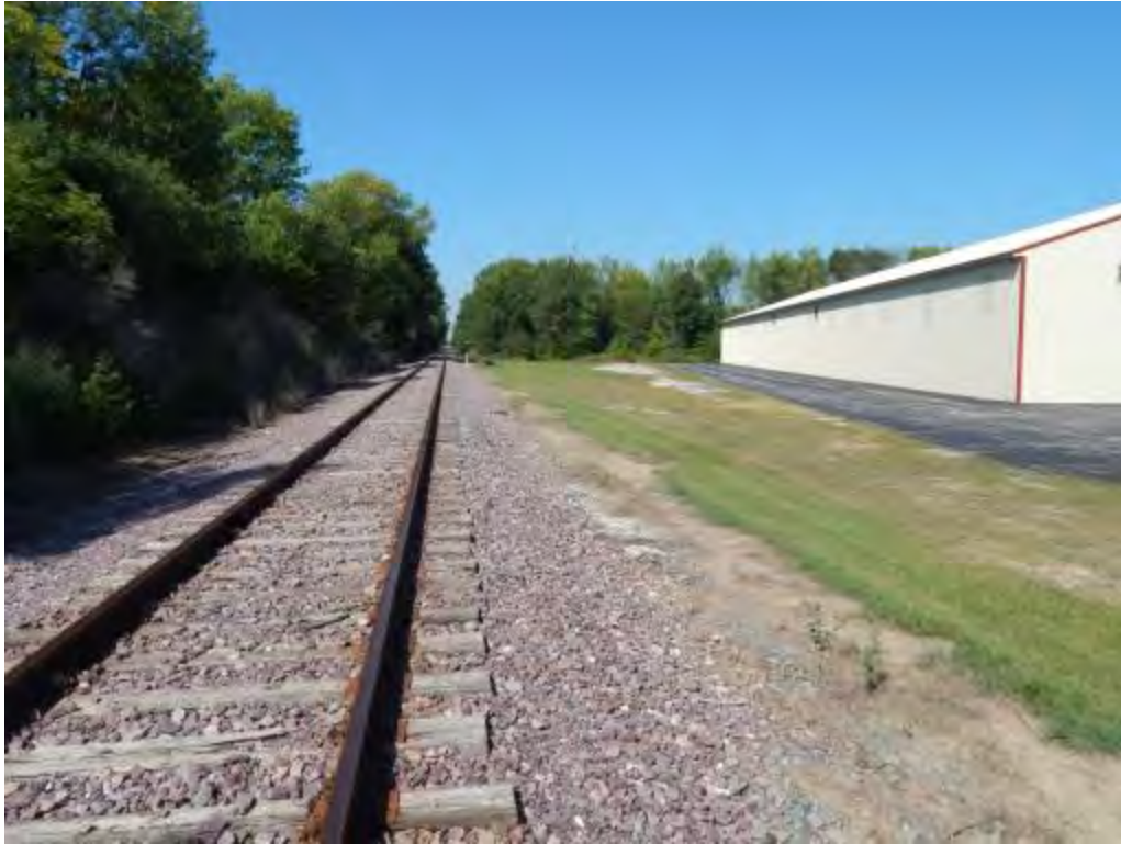
Figure 2-227. Potential Rockwood Spur at WI-310 Transload Location (Looking North) (2014)
