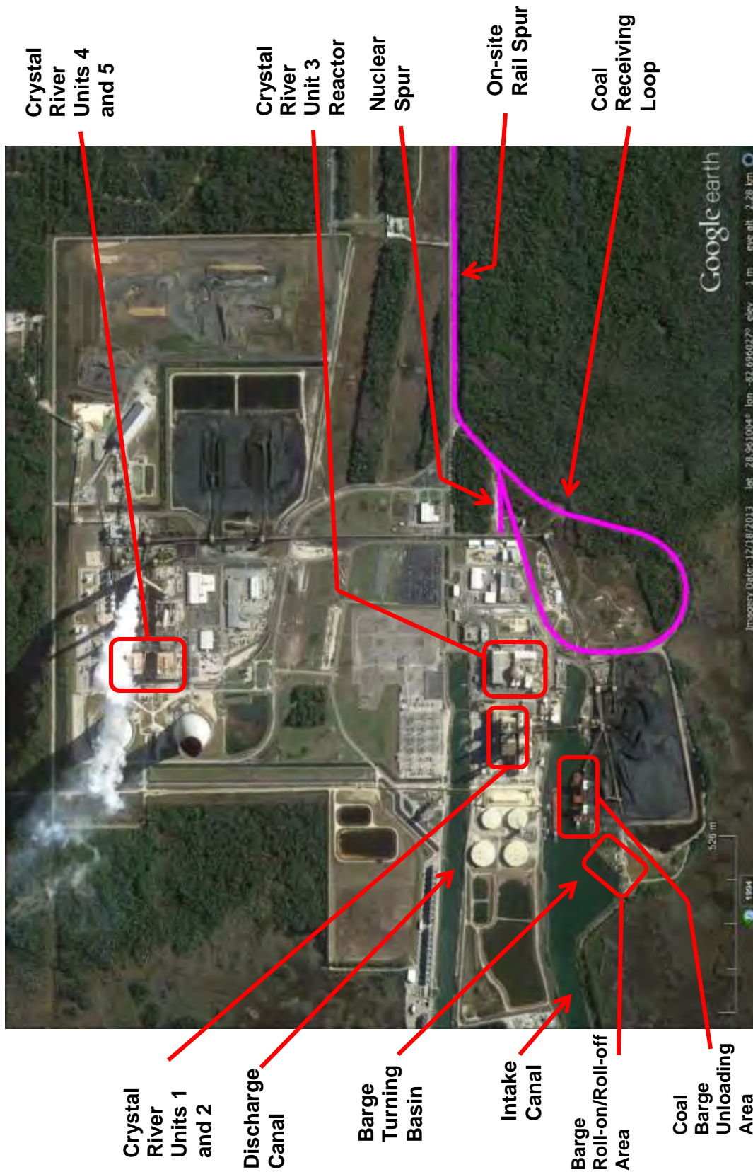
Figure 2-152. Aerial View of the Crystal River Energy Complex (Google 2015)
