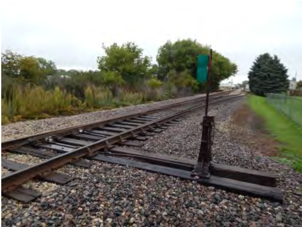
Figure 2-208. Potential Luxemburg Transload Location (Looking East) (2014)
