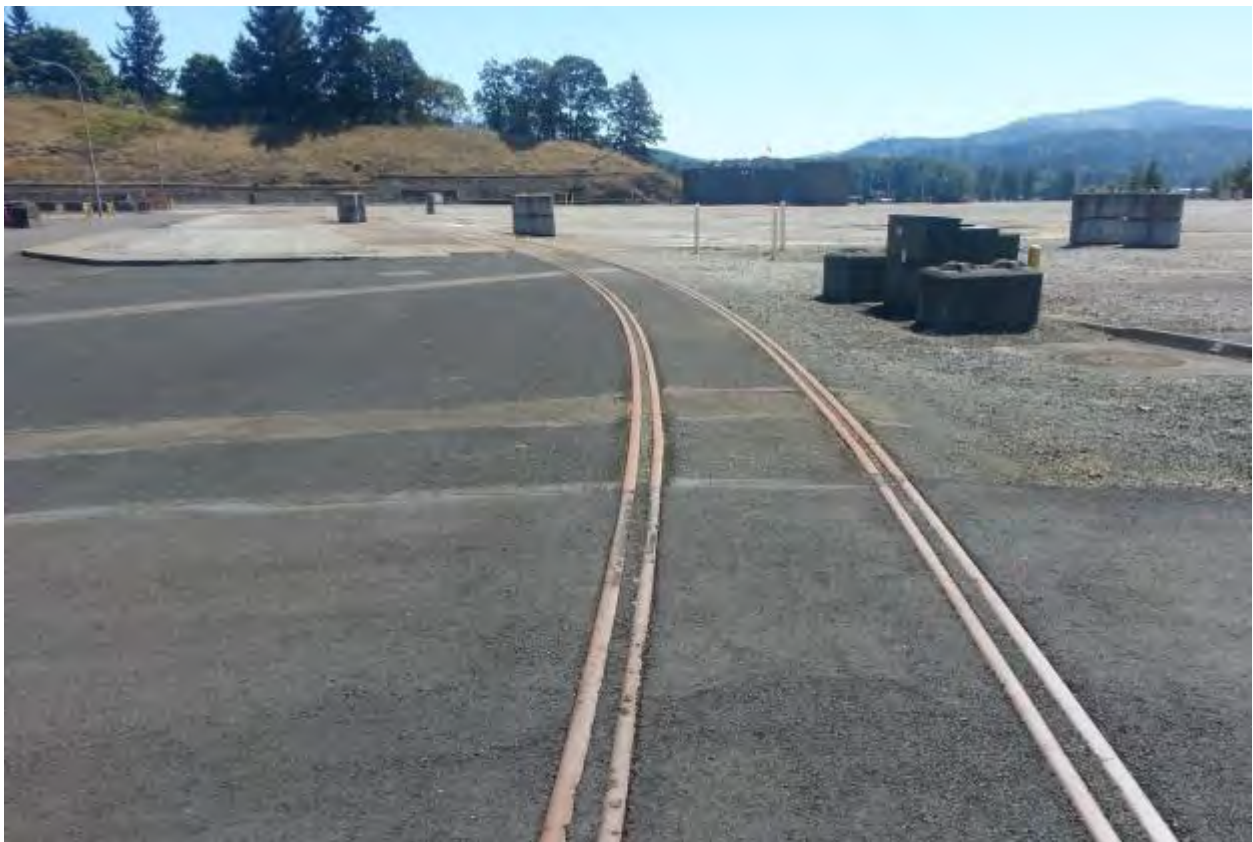
Figure 2-108. Remnants of On-site Rail Spur at Trojan (2013)
