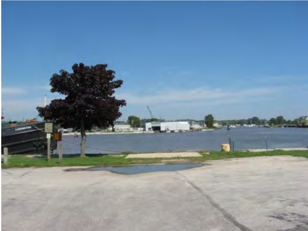
Figure 2-244. Potential Kewaunee Barge Transload Location Parking Lot (2014)
