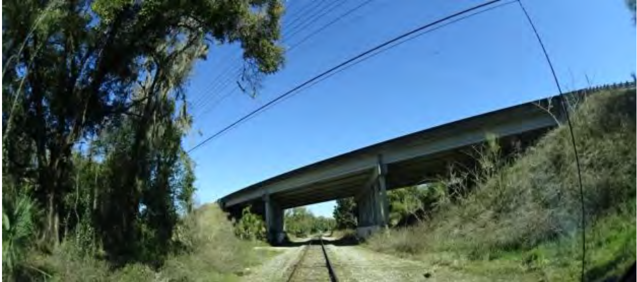
Figure 2-167. Highway Bridge over Florida Northern Railroad (2015)
