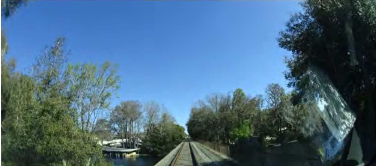
Figure 2-169. Florida Northern Railroad Bridge (2015)
