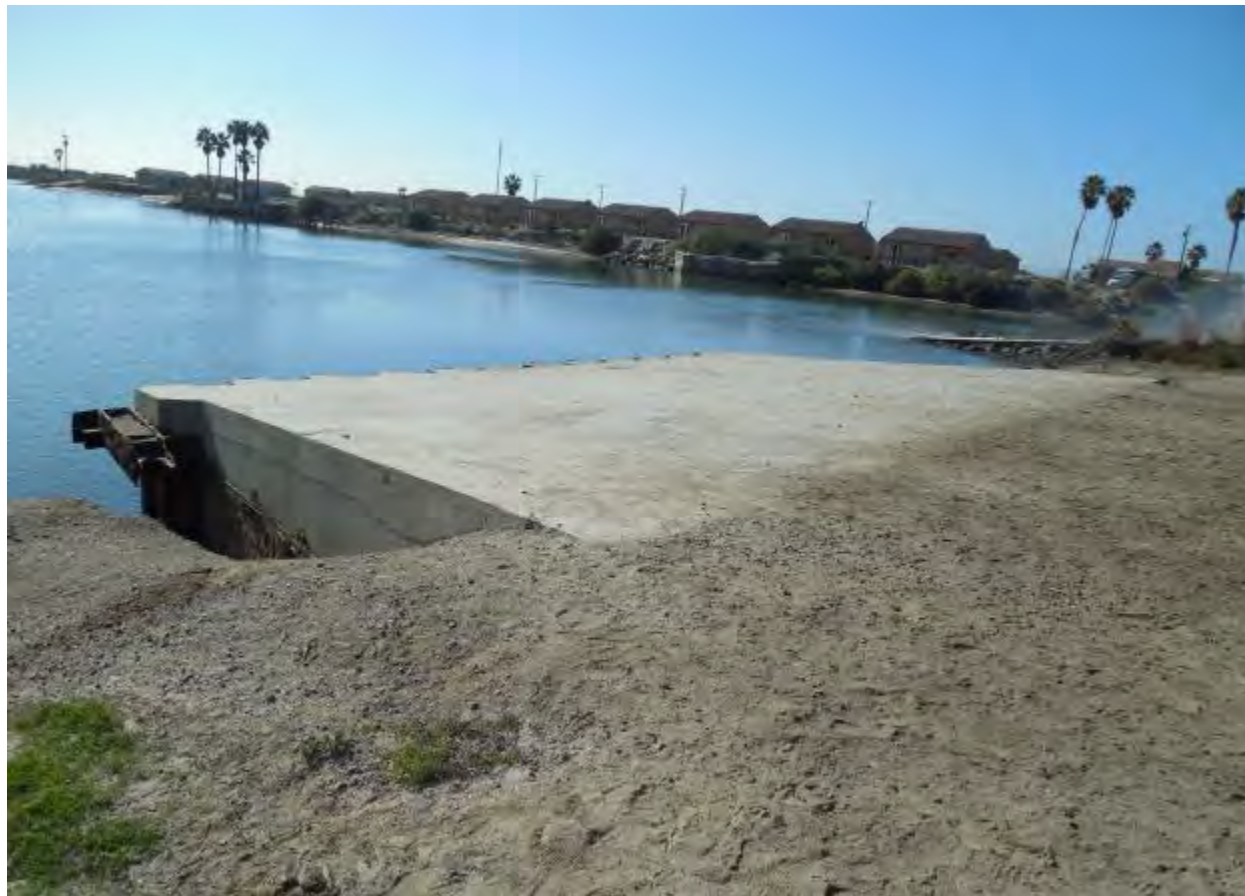
Figure 2-293. Del Mar Boat Basin Bulkhead (2016)
