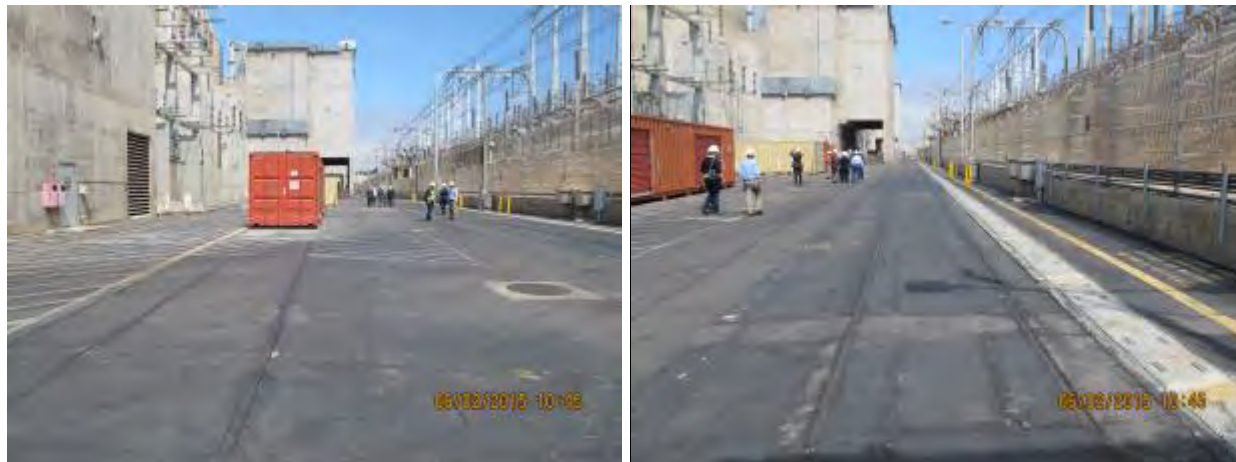
Figure B-52. Site Rail System Looking North (2015)
