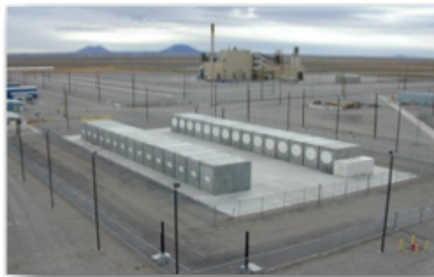
Figure 11. NRC-licensed TMI fuel dry storage in NUHOMS-12T horizontal storage modules at the INL Site.
