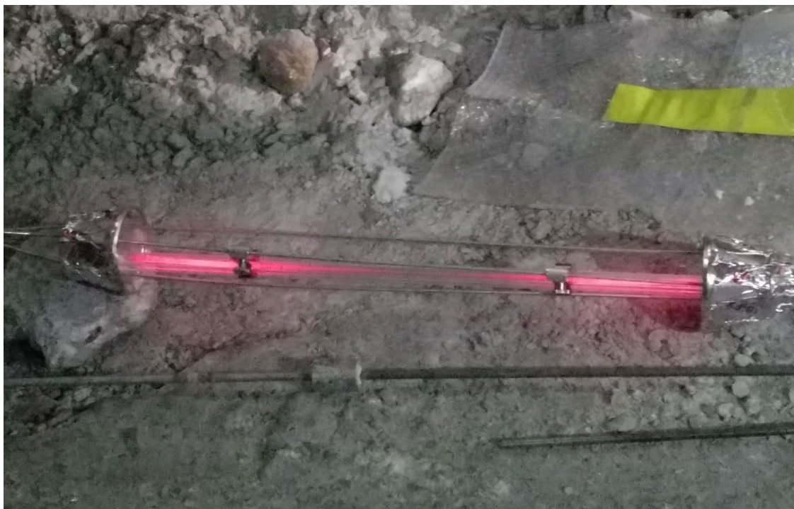
195 196 Figure 2-10: Infrared heater being tested on the floor of the mine at WIPP prior to installation 197
