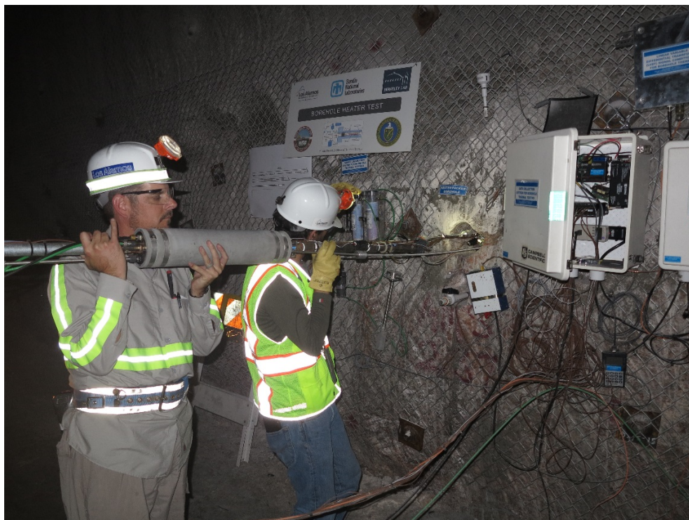
Figure 1-2 Installation of an infrared heater in the WIPP underground.
