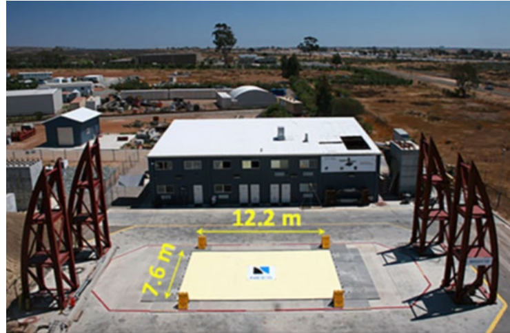
Figure 1-5. LHPOST Outdoor Earthquake Simulator (U.C. San Diego).
