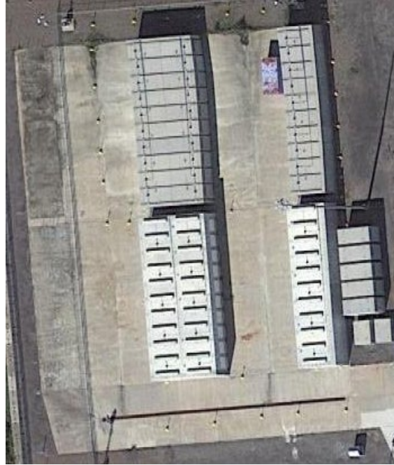
Figure 4-3. Nine Mile Point Nuclear Generating Station ISFSI, Satellite Image from Google Maps, (accessed 6/17/2021).
