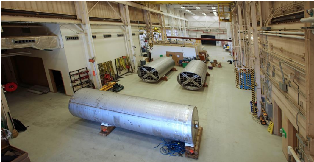
Figure 1.3 Three 32PTH2 spent fuel canisters inside of Sandia's Building 6630 south high bay.
