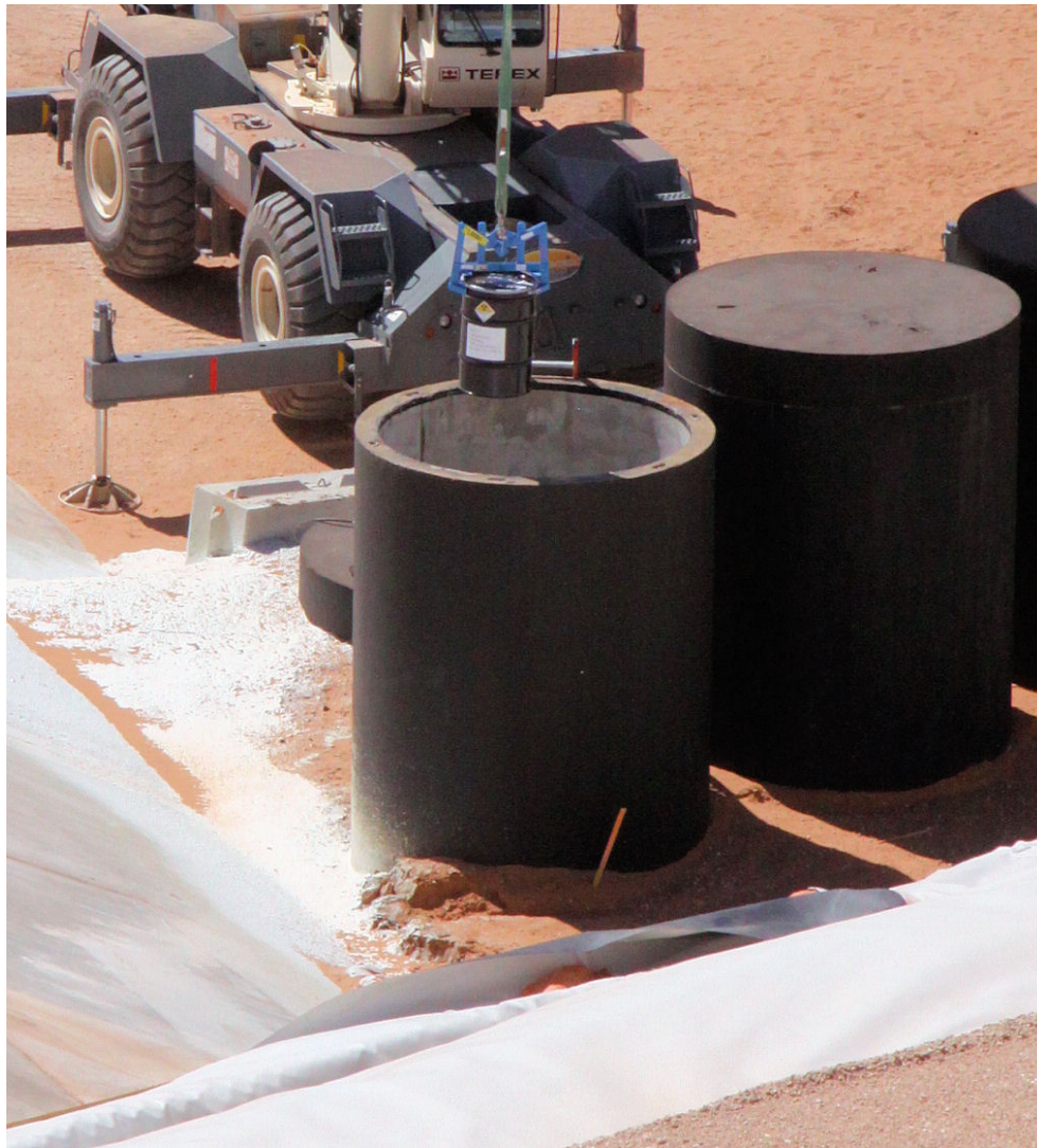
Figure 2-1 Shipment of Sealed Sources is the First Disposal at the Waste Control Specialists Commercial Facility (Courtesy: WCS)
