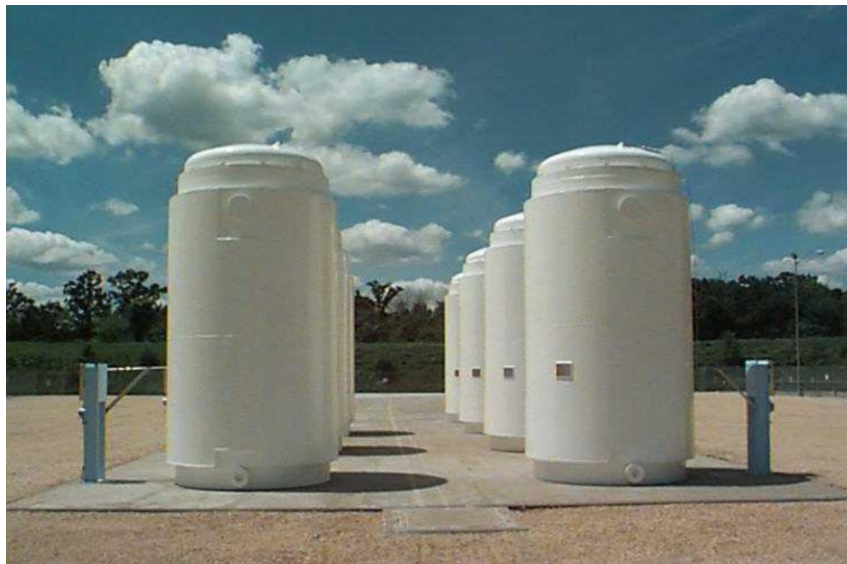
Figure 6-8 Typical Vertical Cask Dry Storage Pad
