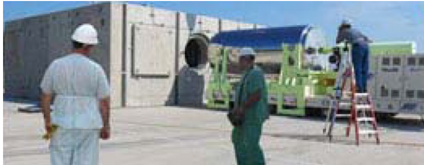
Figure 6-4 Positioning SPMT for Canister Insertion Into A Horizontal Storage Module
