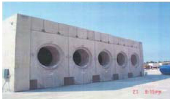
Figure 6-6 Nuhoms Horizontal Storage Unit
