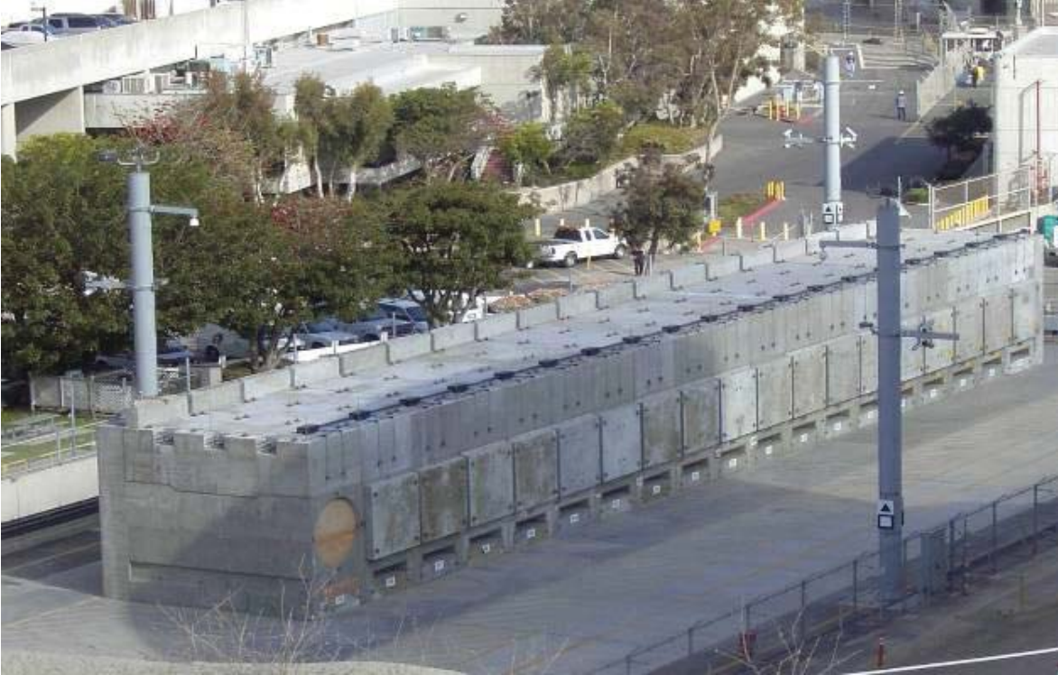
Figure V.1-1: NUHOMS horizontal dry storage systems at San Onofre (Rod McCullum, 2012).
