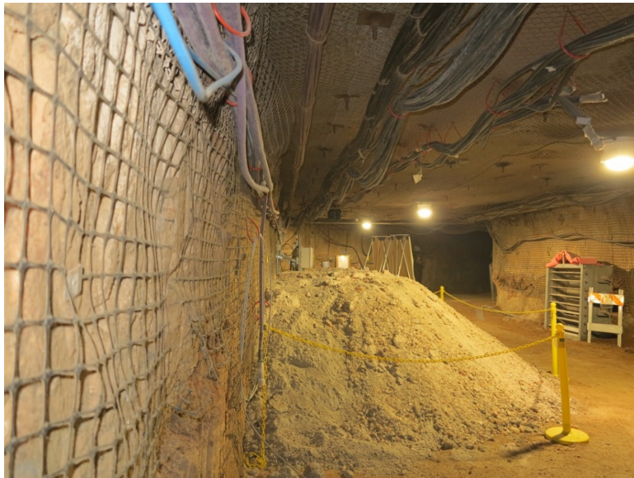
Figure 10: End view of revised schematic, similar to initial schematic but with flattened top of pile extended to wall (top), and constructed ROM salt pile (bottom).
