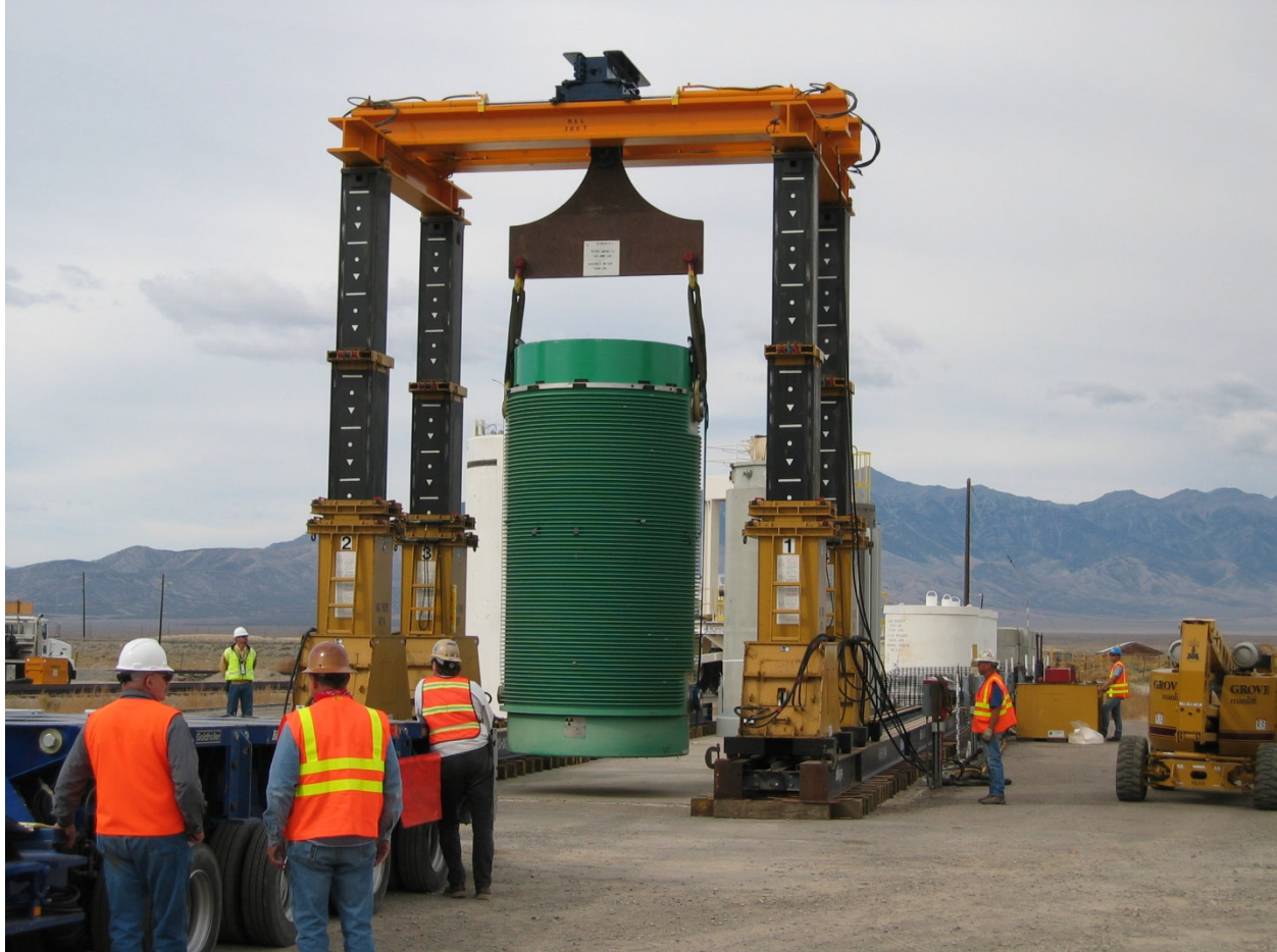
Figure A-3. Hydraulic gantry system lifting the V-21 Cask.
