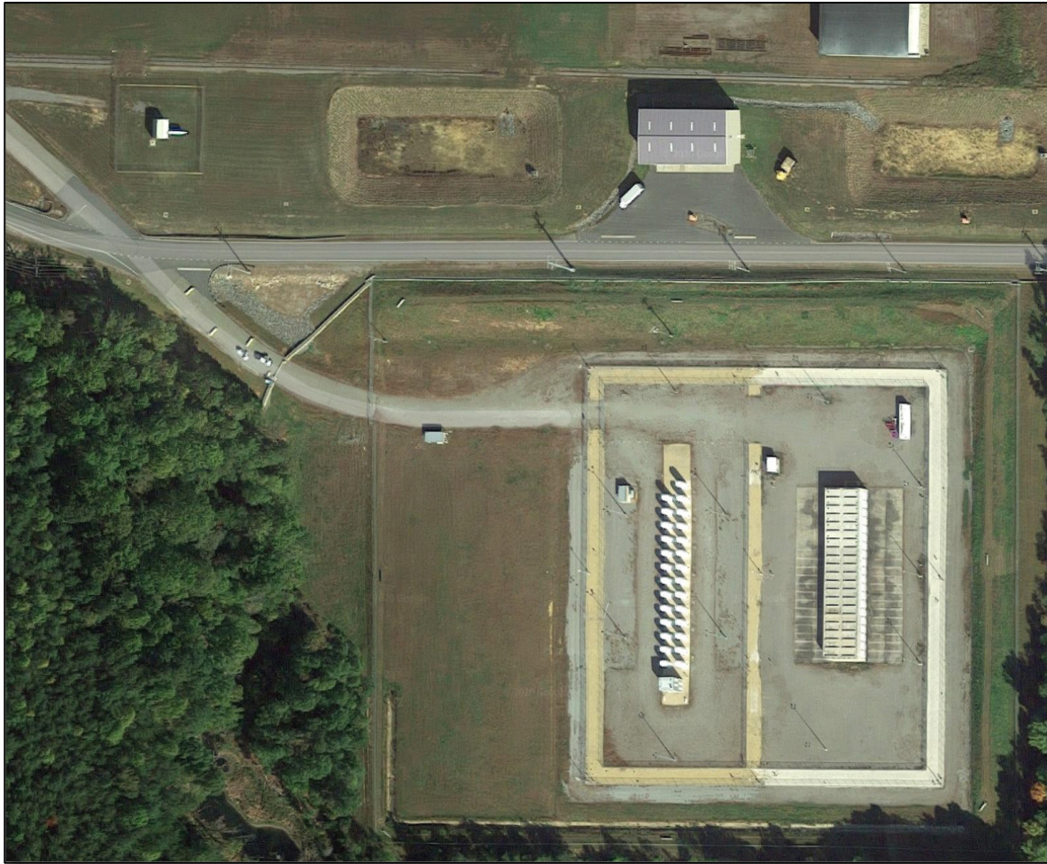
Figure 3. North Anna Power Station ISFSI with Pad 1 on the left (Google Maps screen shot).
