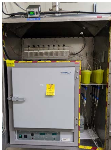
Figure 5. The ventilated canopy housing the oven, effluent taps, and funnels directing leachate to ion exchange columns before proceeding to waste.
