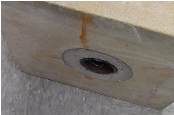
Steel pipe fitted in a block of sandstone
