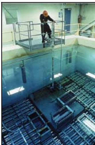
Figure 4.1 Pool Storage at Pickering NGS
