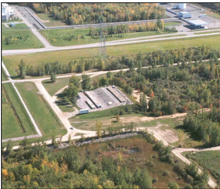
Figure 5.3 Hydro Québec Waste Management Facility
