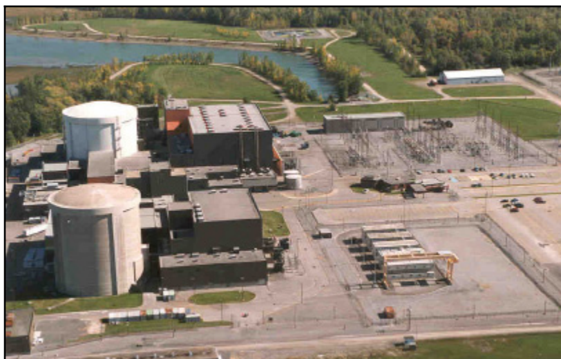
Figure 4.7 Gently-2 Used Fuel Dry Storage Facility – bottom right of picture
