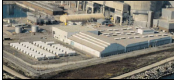
Figure 5.1 PWMF with RCSA on left and Used Fuel Dry Storage Area on right
