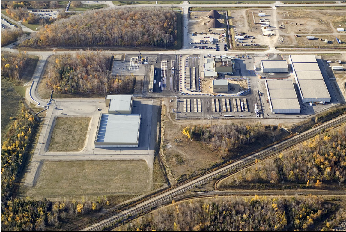
Figure 5.2 Western Waste Management Facility
