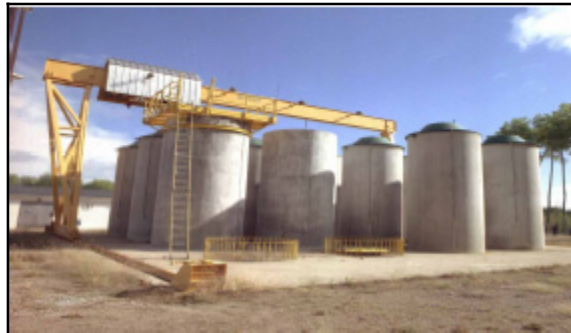
Figure 4.2 AECL Concrete Canisters
