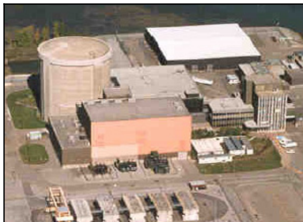
Figure 5.5 Gentilly-1 Waste Management Facility
