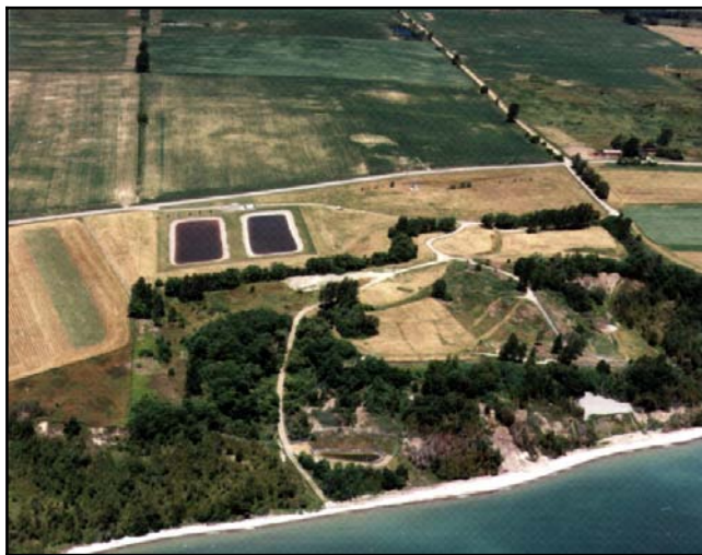
Figure 8.10 – Existing Port Granby Waste Management Facility
