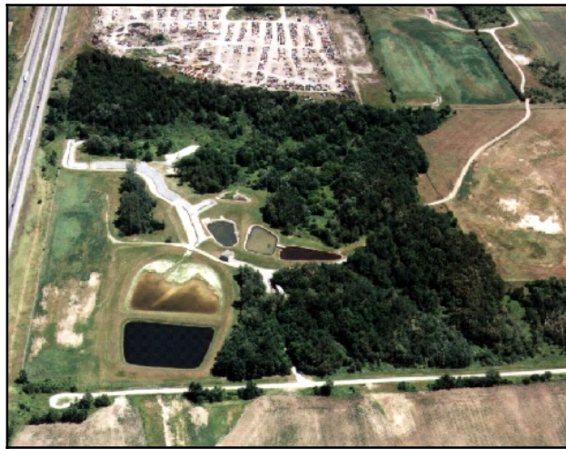
Figure 8.9 – Existing Welcome Waste Management Facility
