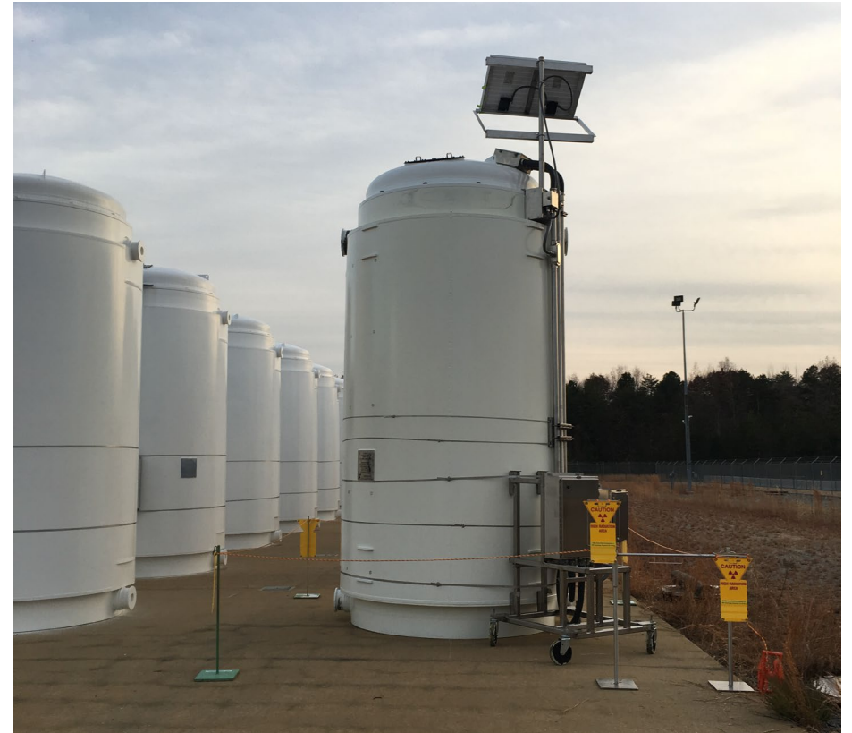
Photo courtesy of Dominion Energy
