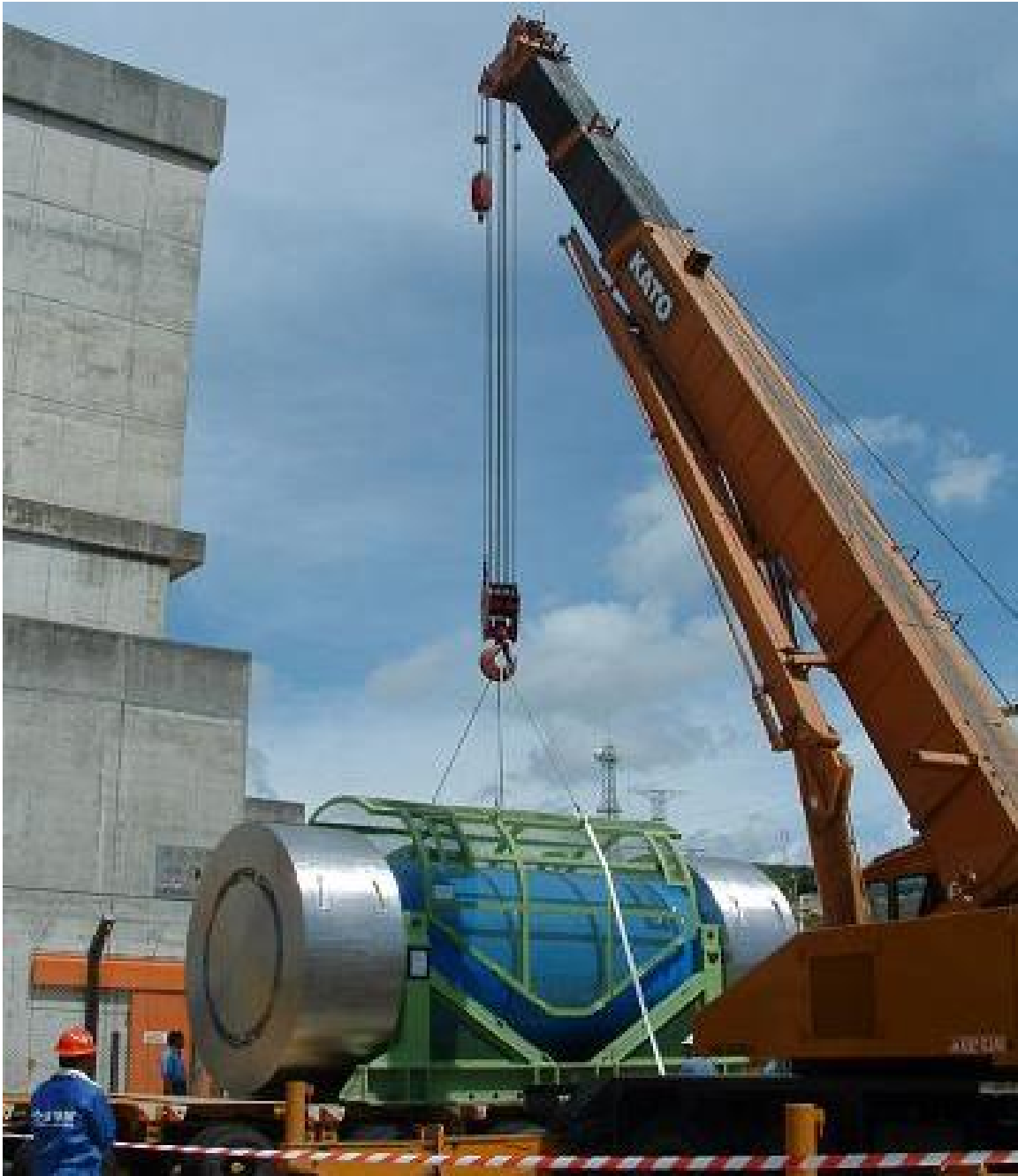
FIGURE 2-25: NAC-STC PACKAGE PERSONNEL BARRIER REMOVAL
