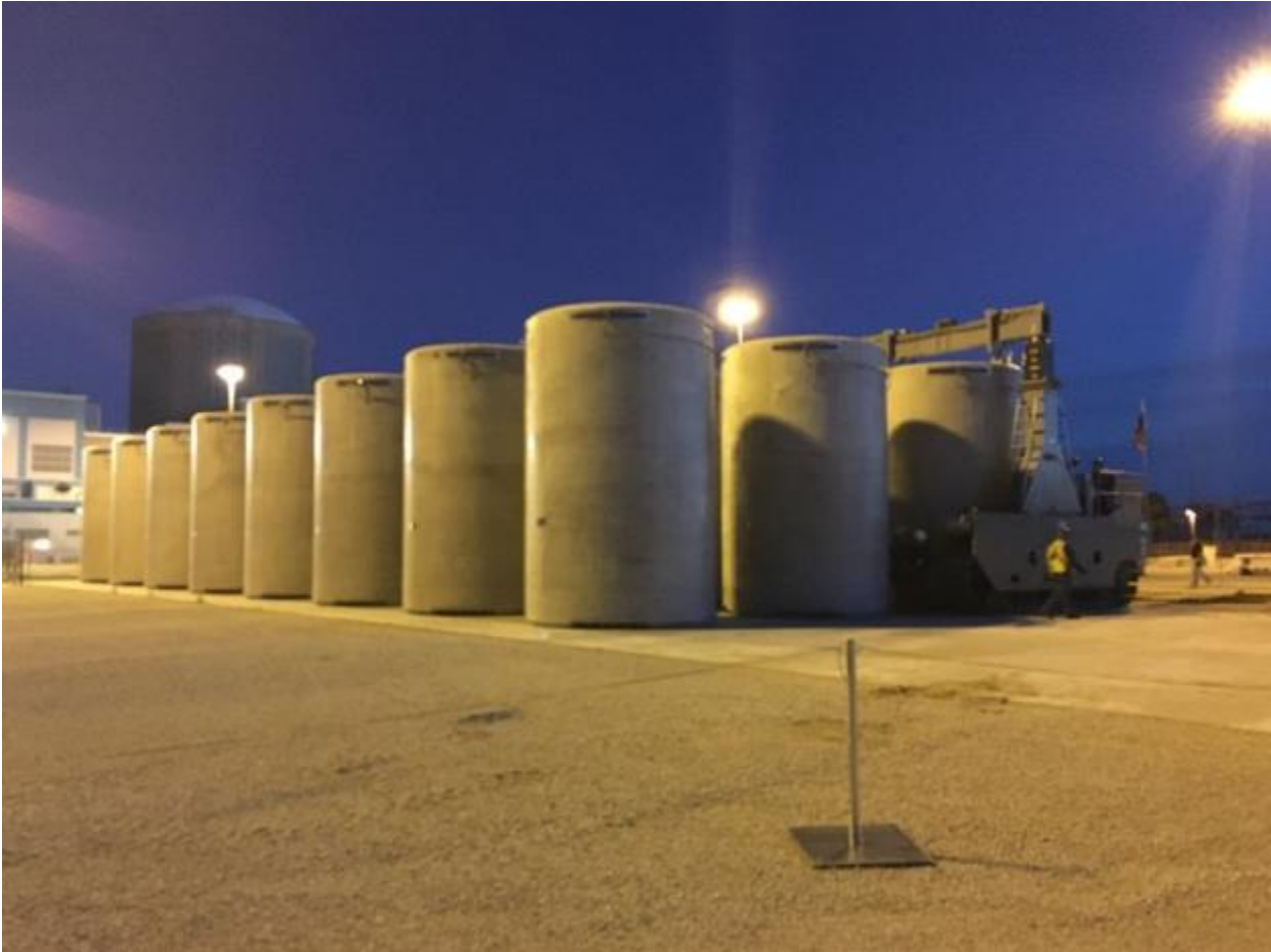
FIGURE 2-17: FINAL LOADED MAGNASTOR VERTICAL CONCRETE CASK (CC4) [19] POSITIONED ON KPS ISFSI PAD
