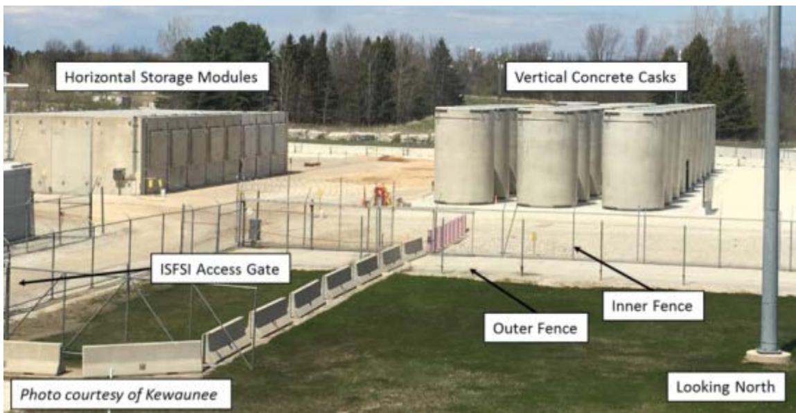
FIGURE 2-5: KEWAUNEE ISFSI STORAGE CASKS
