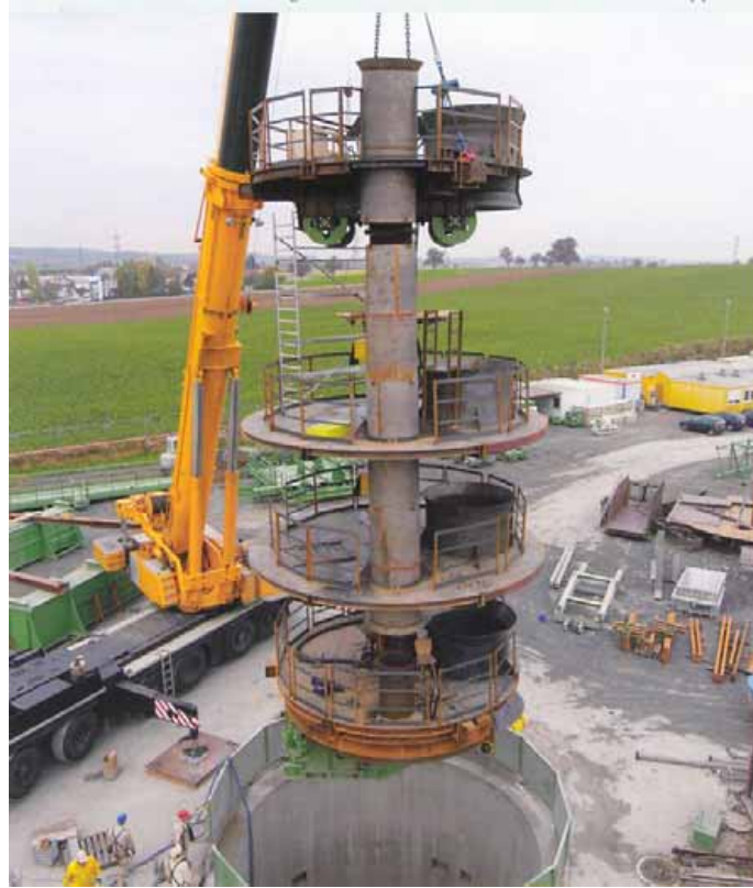
Figure 7.5.1 Shaft sinking platform (salt mine of Konradsberg – Heilbronn – Germany)
