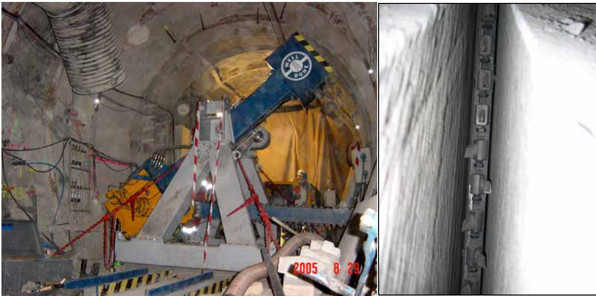
Figure 7.7.5 Groove excavation for the KEY test at the Meuse/Haute Marne laboratory
