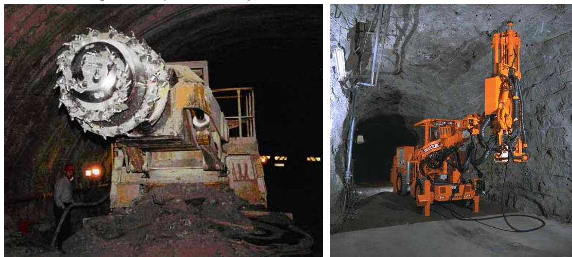
Figure 5.1.22 Examples of roadheader and bolting jumbo
