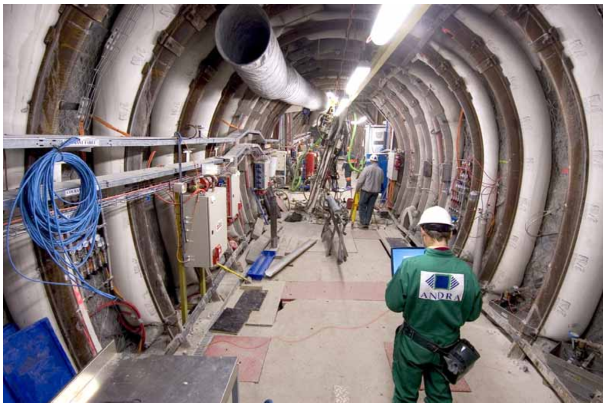
Figure 2.3.5 View of the Meuse/Haute-Marne underground research laboratory drift at -445 m
