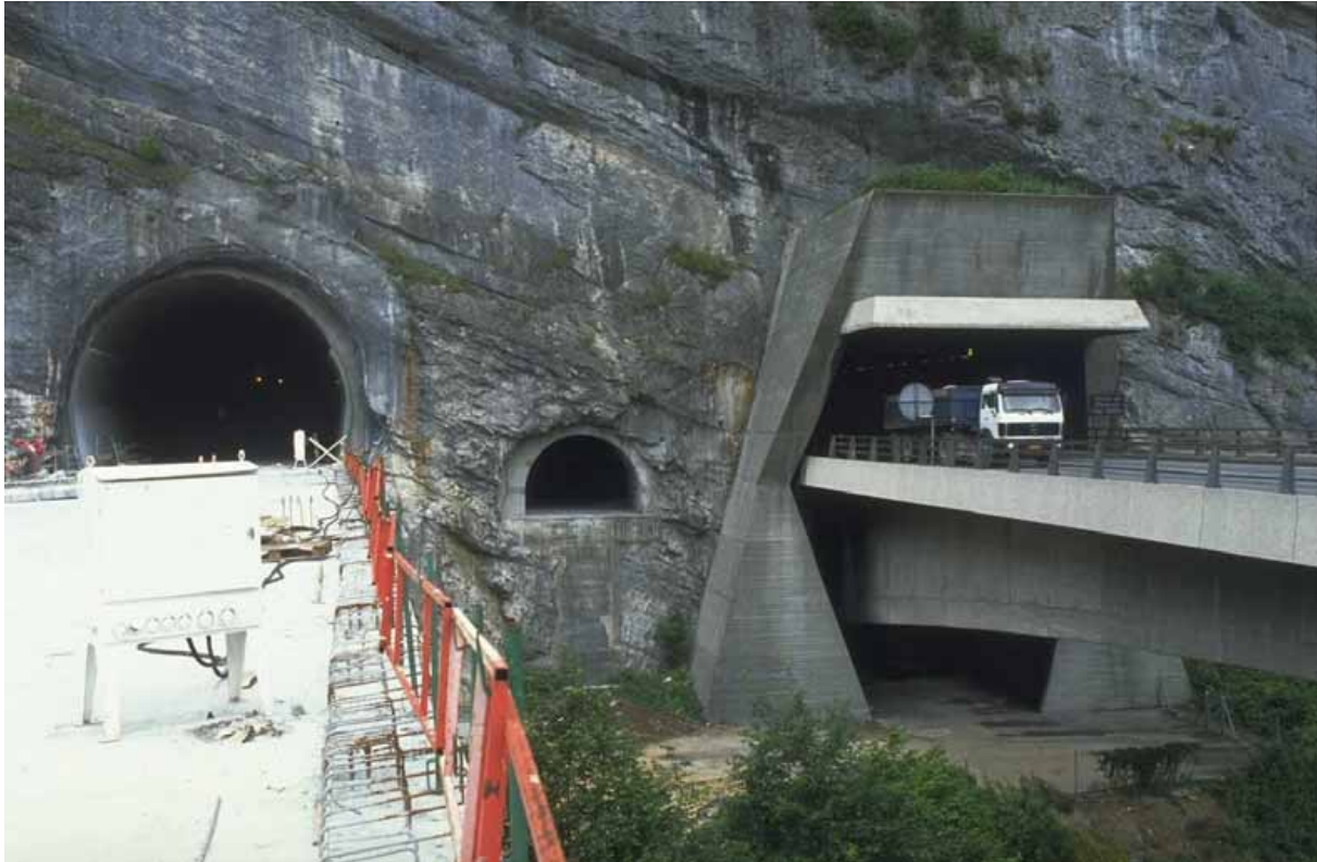
Figure 2.3.4 Entrance to the Chamoise tunnel (left, tube under construction; centre, exploratory drift; right, tube in operation)
