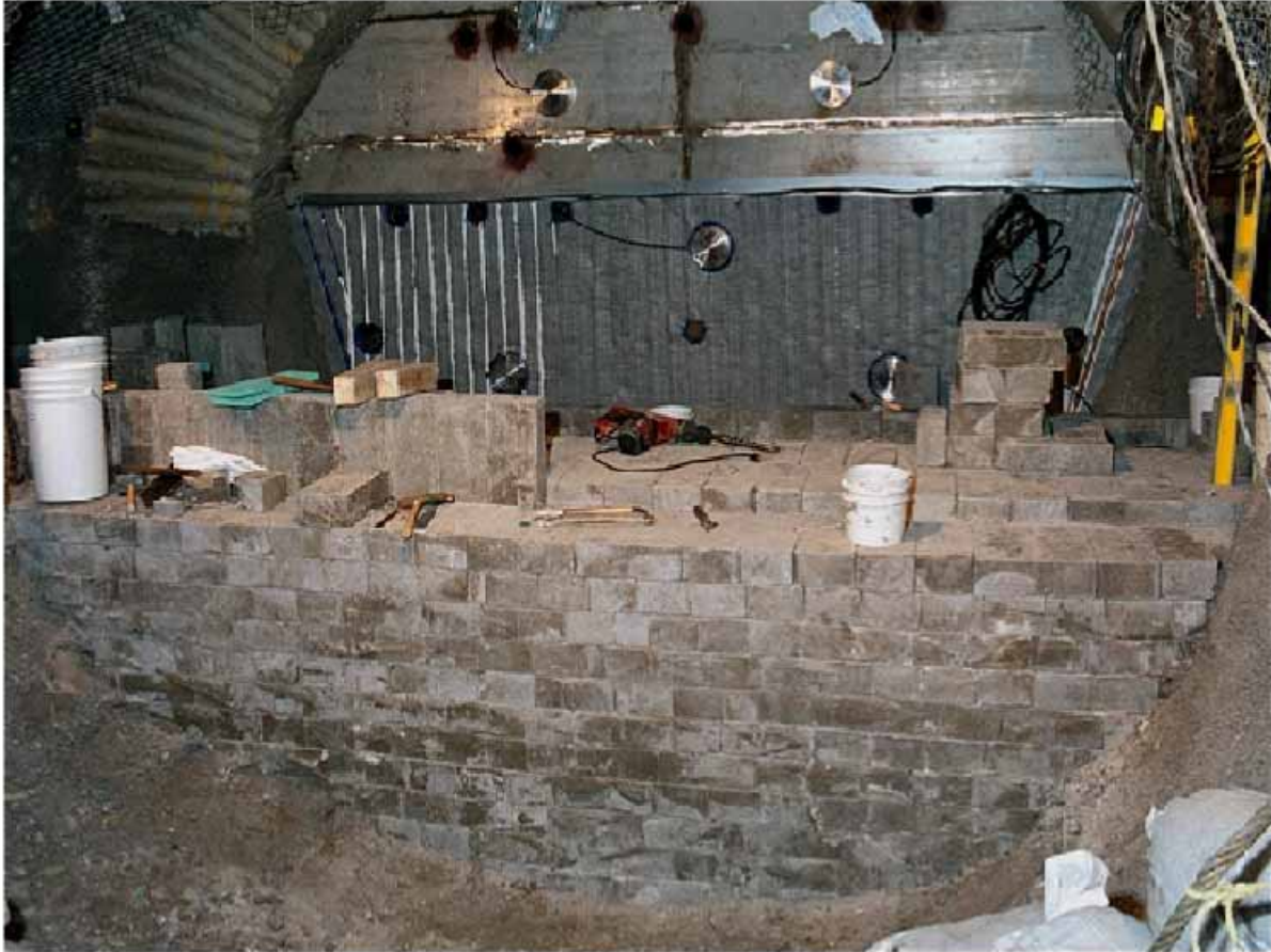
Figure 7.7.4 Experimental seal made up of bentonite blocks - Tunnel Sealing Experiment in Canada (these blocks would be larger at industrial scale).
