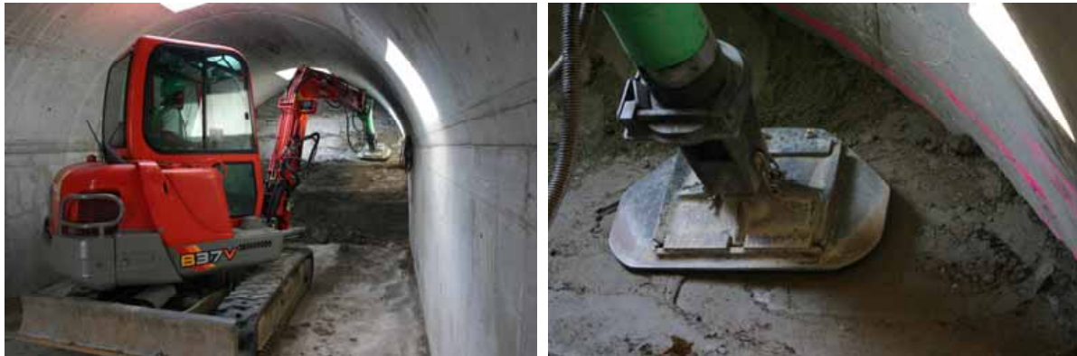
Figure 7.7.1 Hydraulic ram in action in the backfill demonstration model
