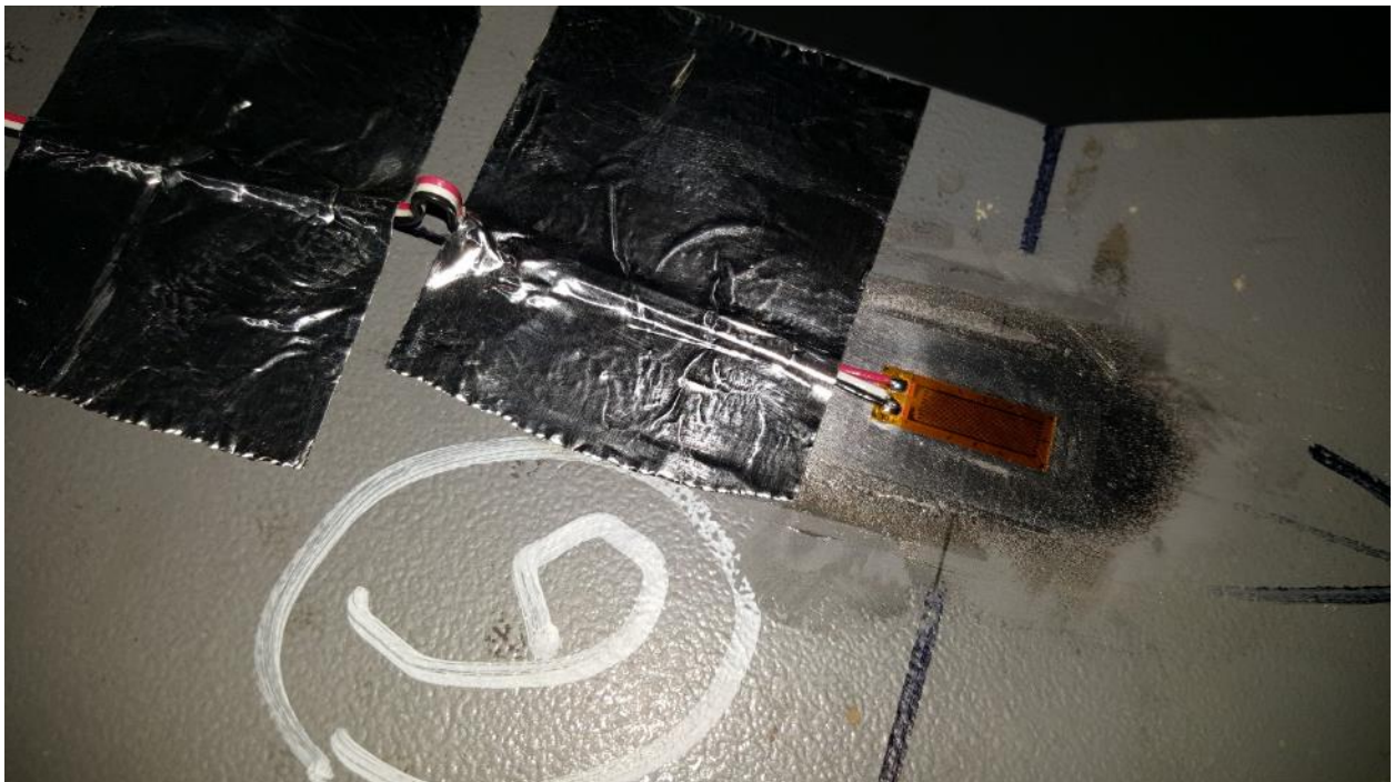
Figure D10. SGBF6 Front of Bottom Flange of #4 Cross Bearer, LH Side between Center Sill and Side Sill, near Center Sill
