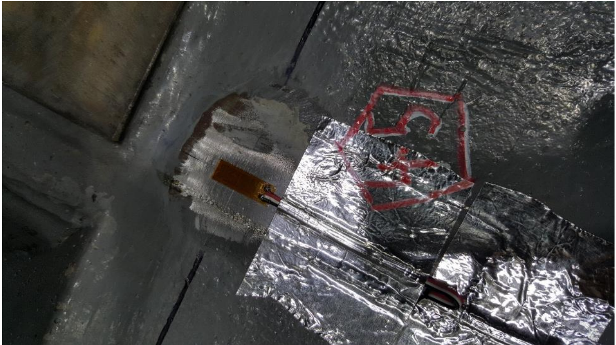
Figure D49. SGBF45 Top of Deck Plate, above LH Side Sill Web, approximately 2" aft of #2 Cross Bearer
