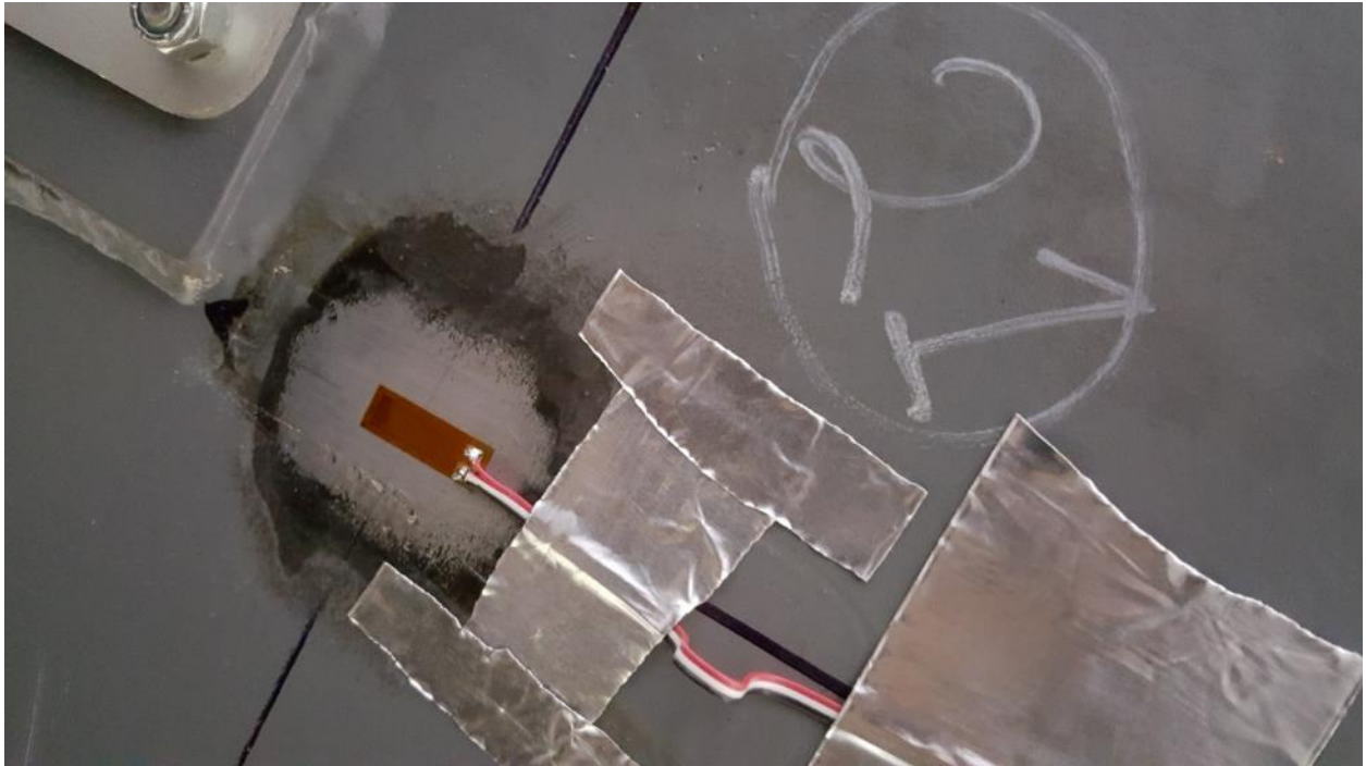
Figure D25. SGBF21 Center Sill Bottom Flange, aligned with LH Center Sill Web, at Longitudinal center of Car
