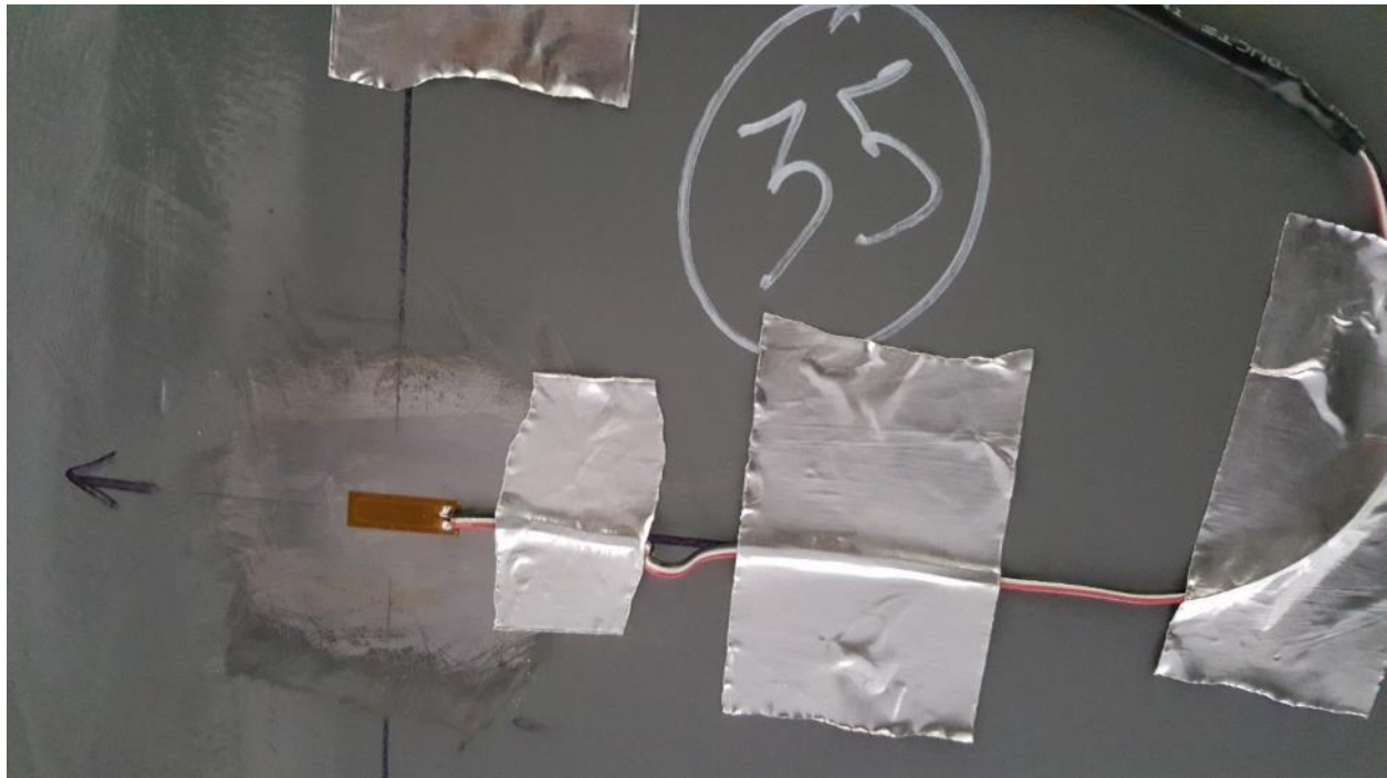
Figure D39. SGBF35 RH Side of Bottom Flange of Center Sill, forward of Rear Body Bolster, aligns with Center Sill Web and End Stop Mount Block Pin Hole
