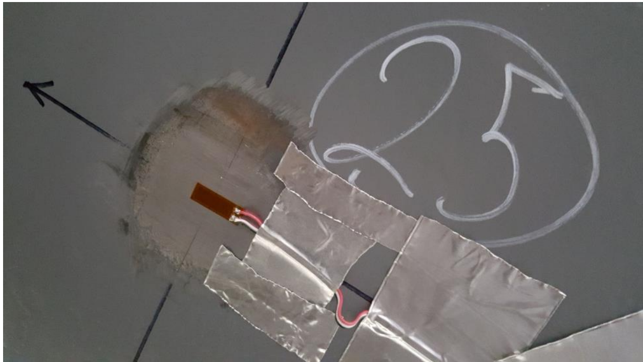
Figure D29. SGBF25 Center Sill Bottom Flange, aligned with LH Center Sill Web, approximately 2" aft of #2 Cross Bearer
