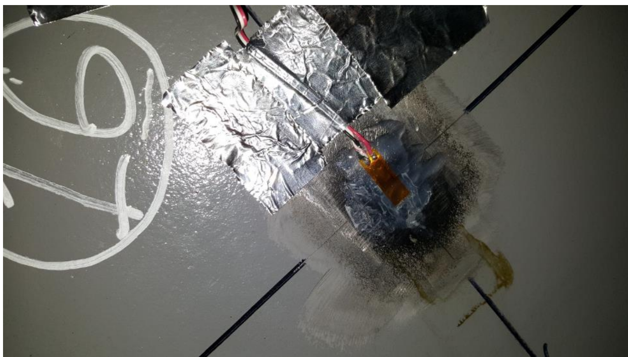
Figure D20. SGBF16 Center Sill Bottom Flange, aligned with RH Center Sill Web, approximately 2" forward of #3 Cross Bearer
