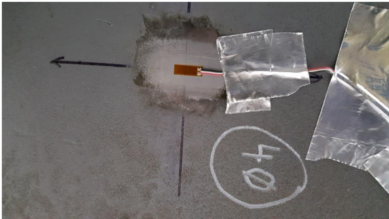
Figure D44. SGBF40 Rear of Bottom Flange of Rear Body Bolster near Center Sill, LH Side
