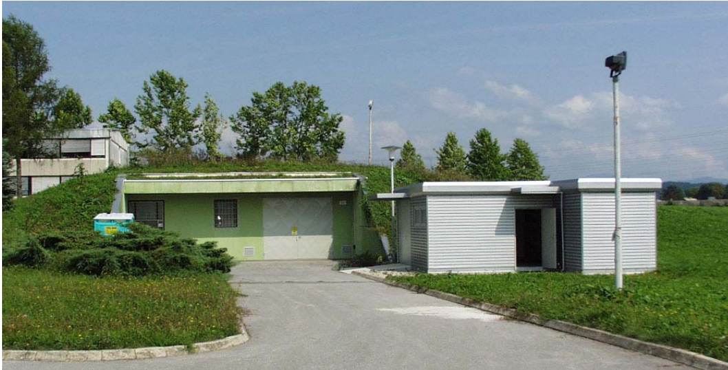
Figure 4. Central interim storage facility for radioactive waste from small producers
