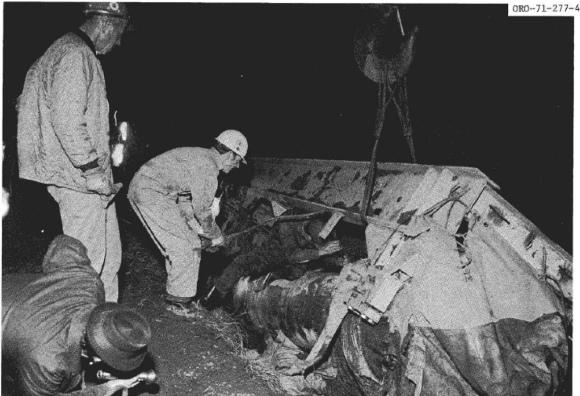
Fig. 4-4. Initial lift during cask retrieval (Chandler 1972).
