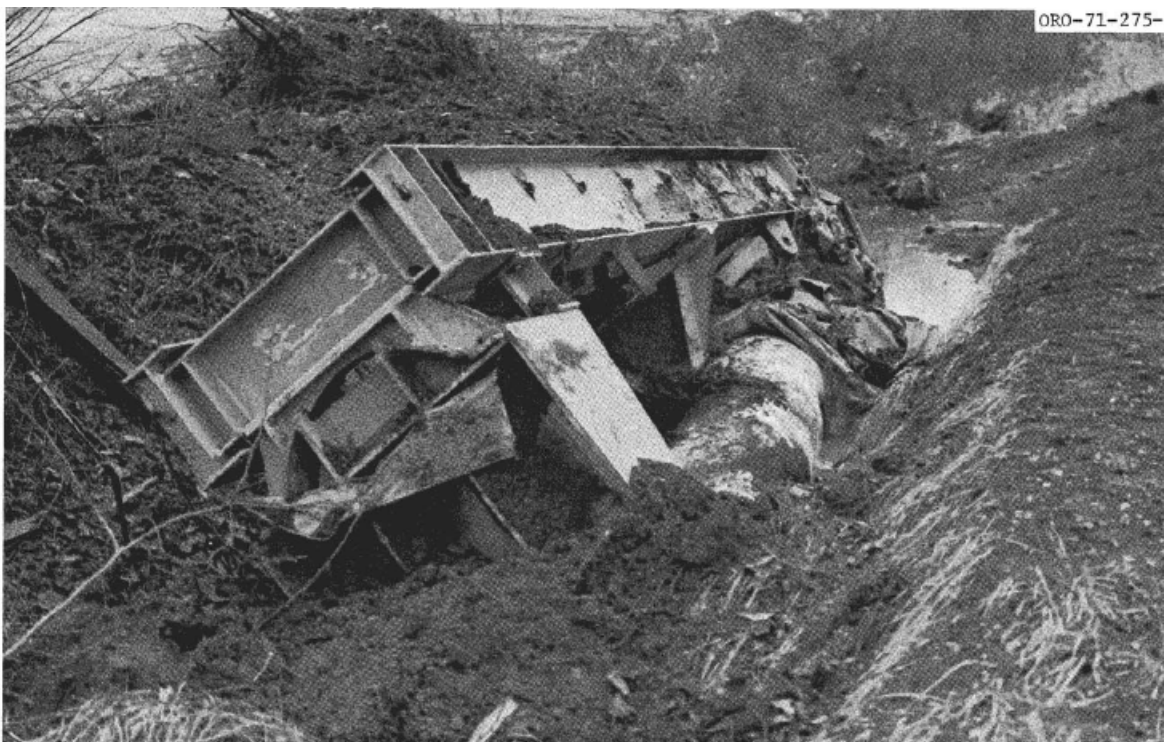
Fig. 4-1. Hallam cask embedded in ditch with skid after accident (Chandler 1972).
