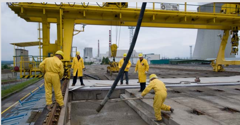
The pouring of concrete over an emplacement vault.
