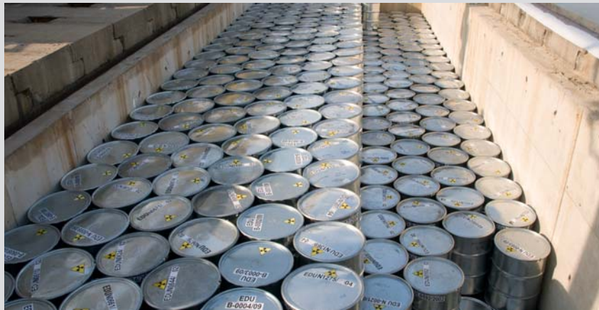
Radioactive waste storage in an emplacement chamber.
