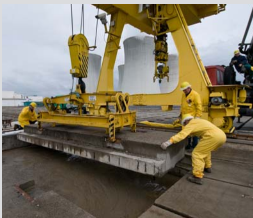
Covering the vault with panels.
