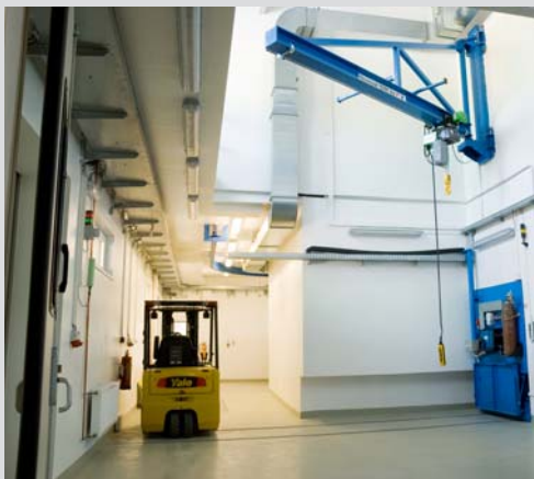
Hall in the operations building.
