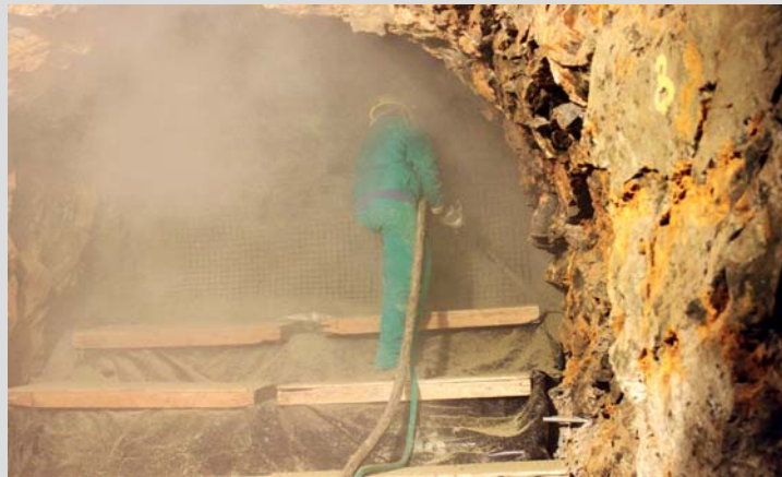
Experimental research of shotcrete backfill technology.
