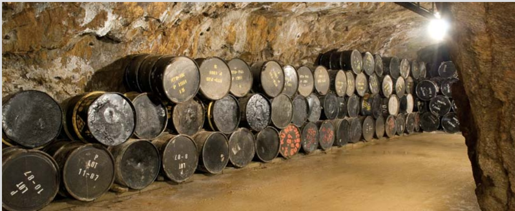
Radioactive waste in an emplacement chamber at the Bratrství repository.
