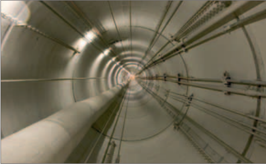
Access shaft of the Meuse/Haute-Marne underground research laboratory
