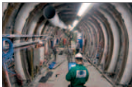
Experimental drift (~ 445 metres) of the Meuse/Haute-Marne laboratory
