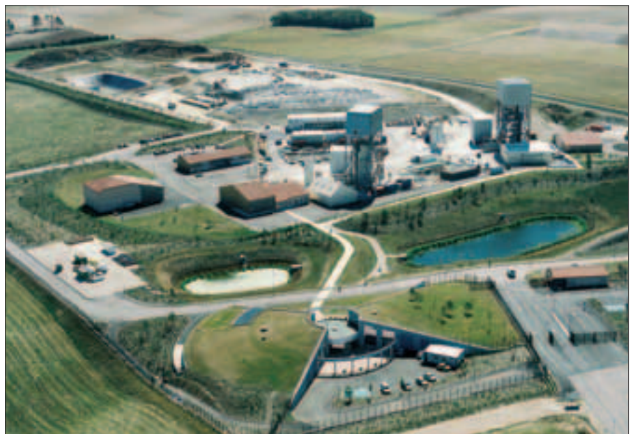
Aerial view of the Meuse/Haute-Marne underground research laboratory
