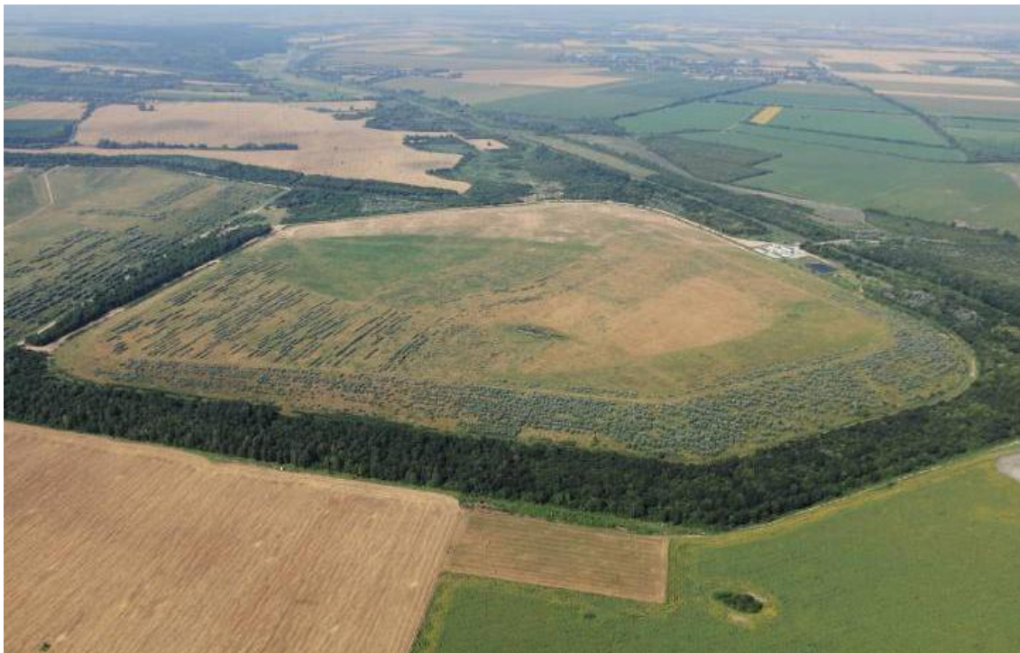
Remediated uranium industry sludge store
