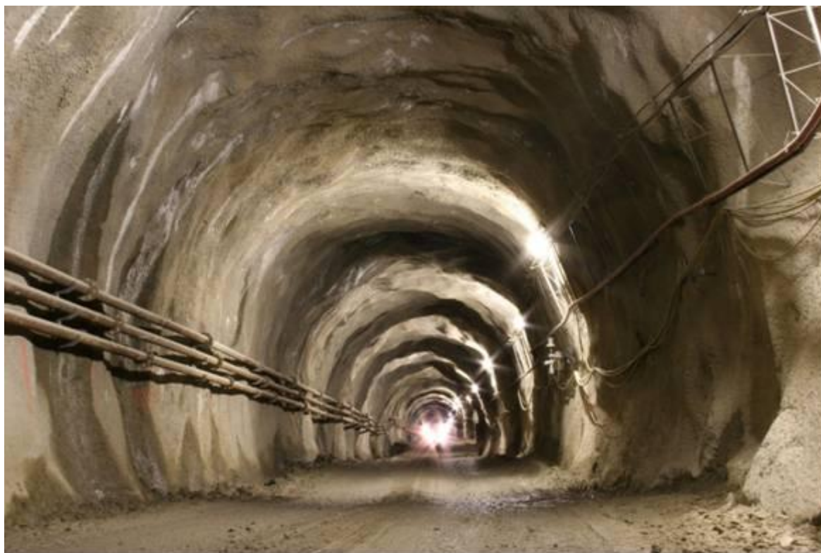
Eastern underground declined shaft of National Radioactive Waste Repository
