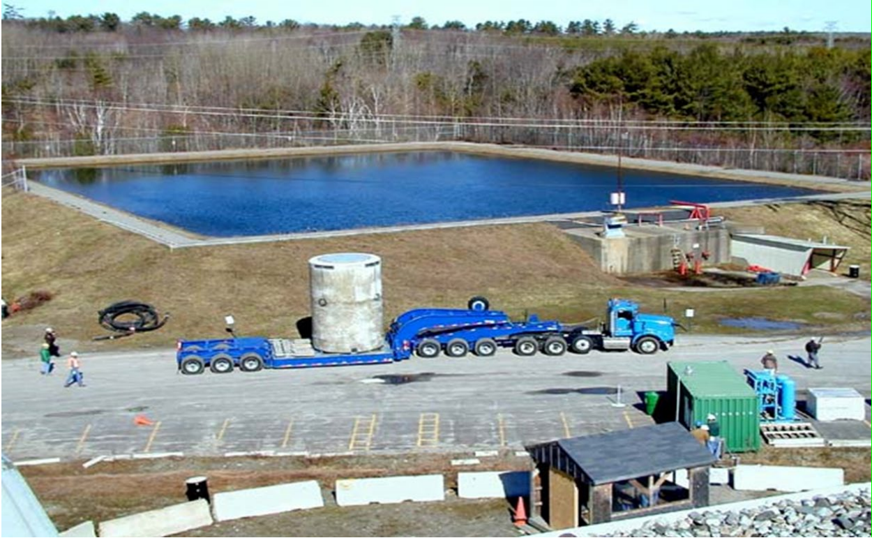
Figure 2-25: Loaded VCC on HHT
