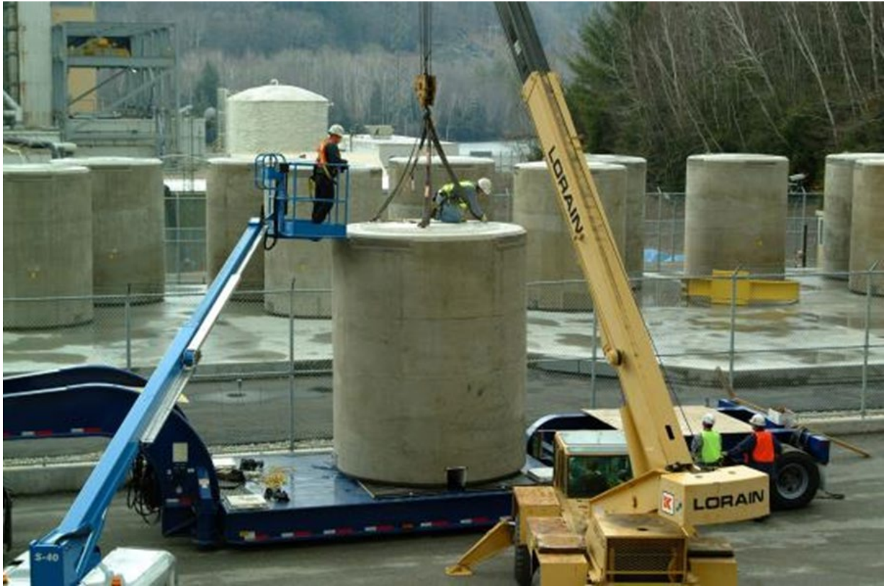
Figure 2-26: VCC Lid Installation on VCC Positioned on HHT
