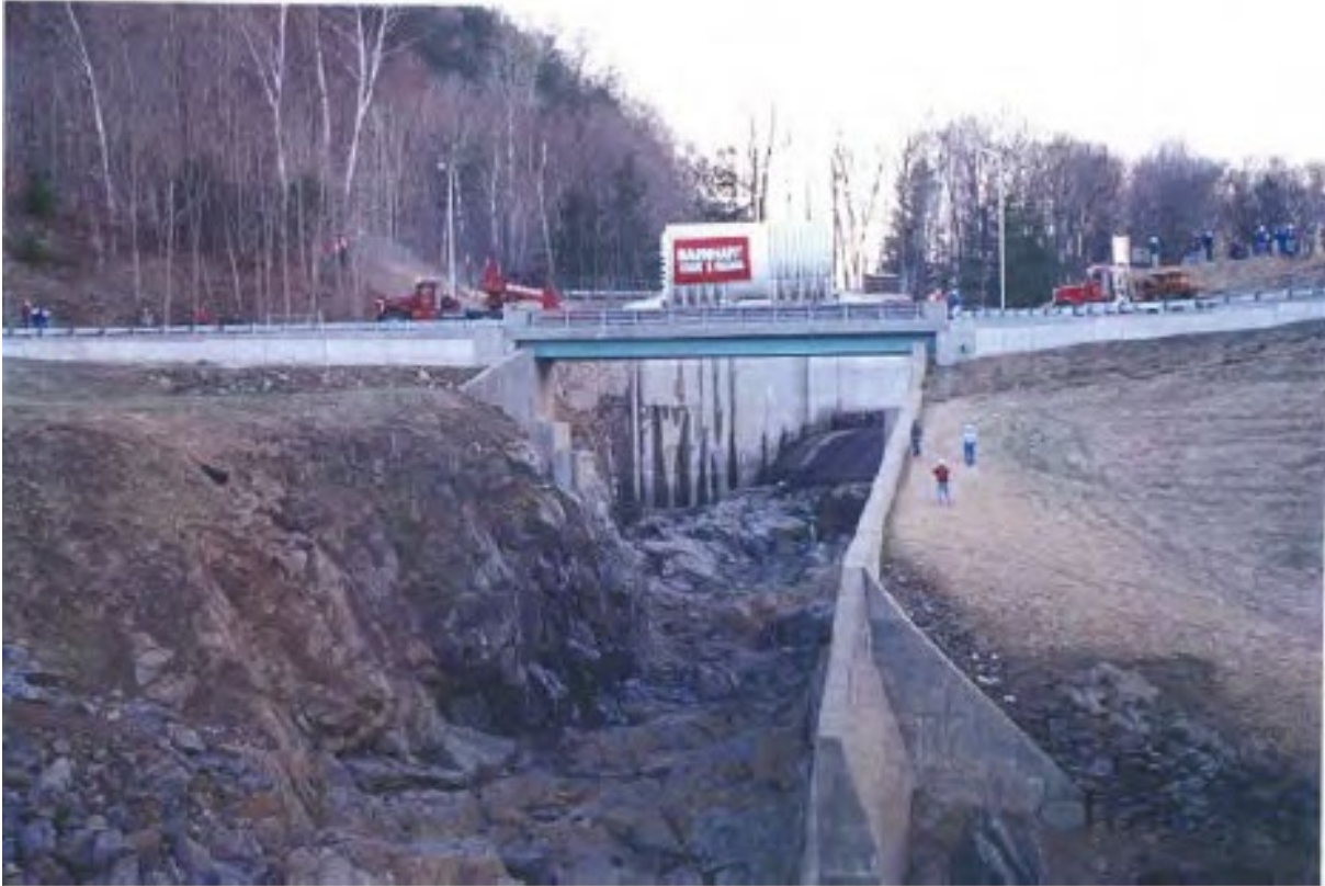
Figure 2-9: Spillway Bridge on Sherman Dam (1997) [5]
