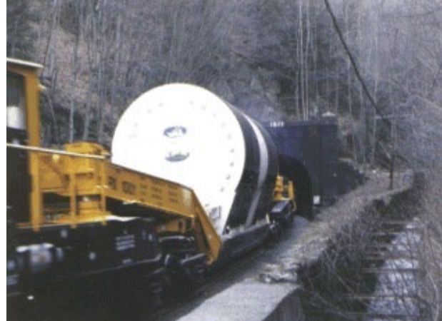
Figure 3-15: Removal of YR Pressure Vessel
