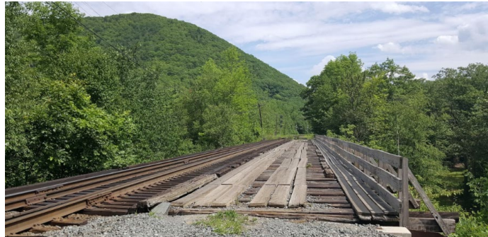
Figure 3-16: Track across bridge to the East of Hoosac Tunnel [51]
