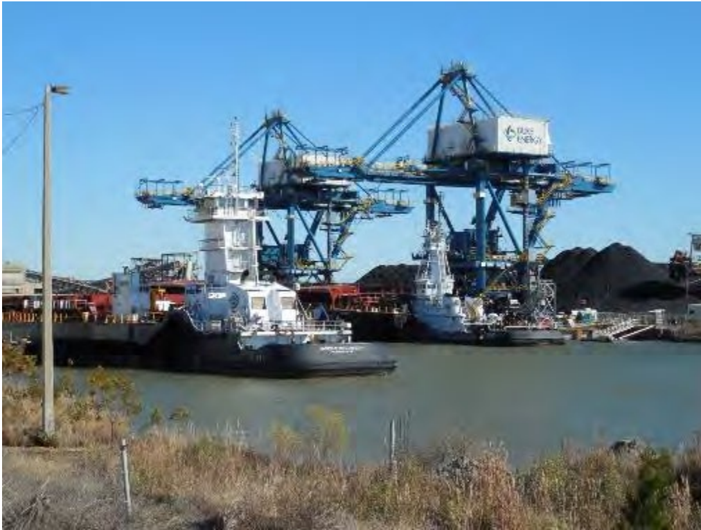
Figure 2-18: Current Barge Area Used for Unloading Coal Barges [2]
