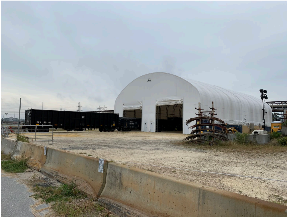
Figure 2-11: Big Top Tent at end of Nuclear Spur [55]
