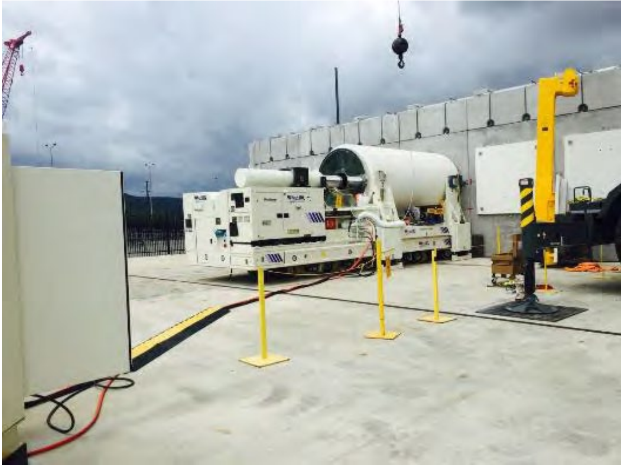
Figure 2-5: Transfer Cask being Used to Load Canister into HSM [2]
