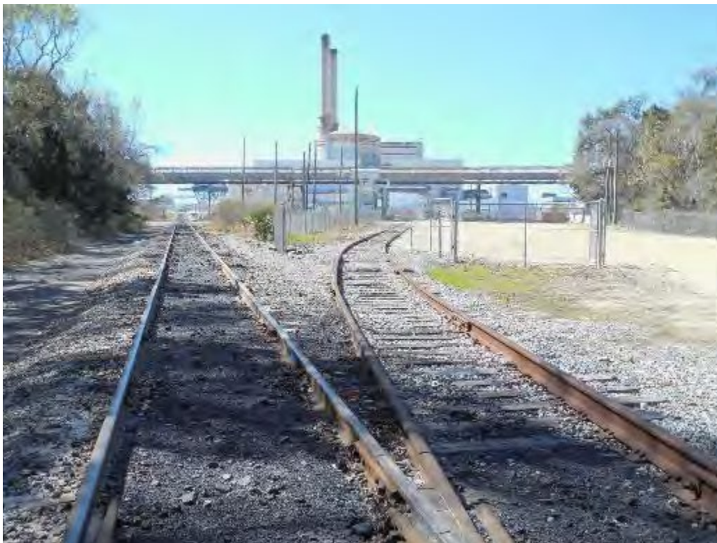
Figure 2-12: Junction of On-Site Industrial Spur (left) and Nuclear Spur (right) [2]
