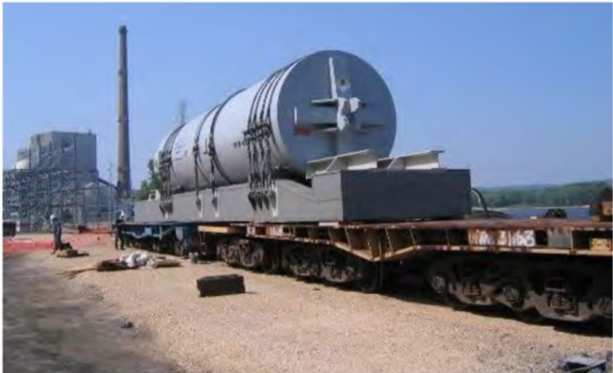
Figure 3-1: LACBWR Reactor Pressure Vessel on the LACBWR Rail Spur (2007) [7]
