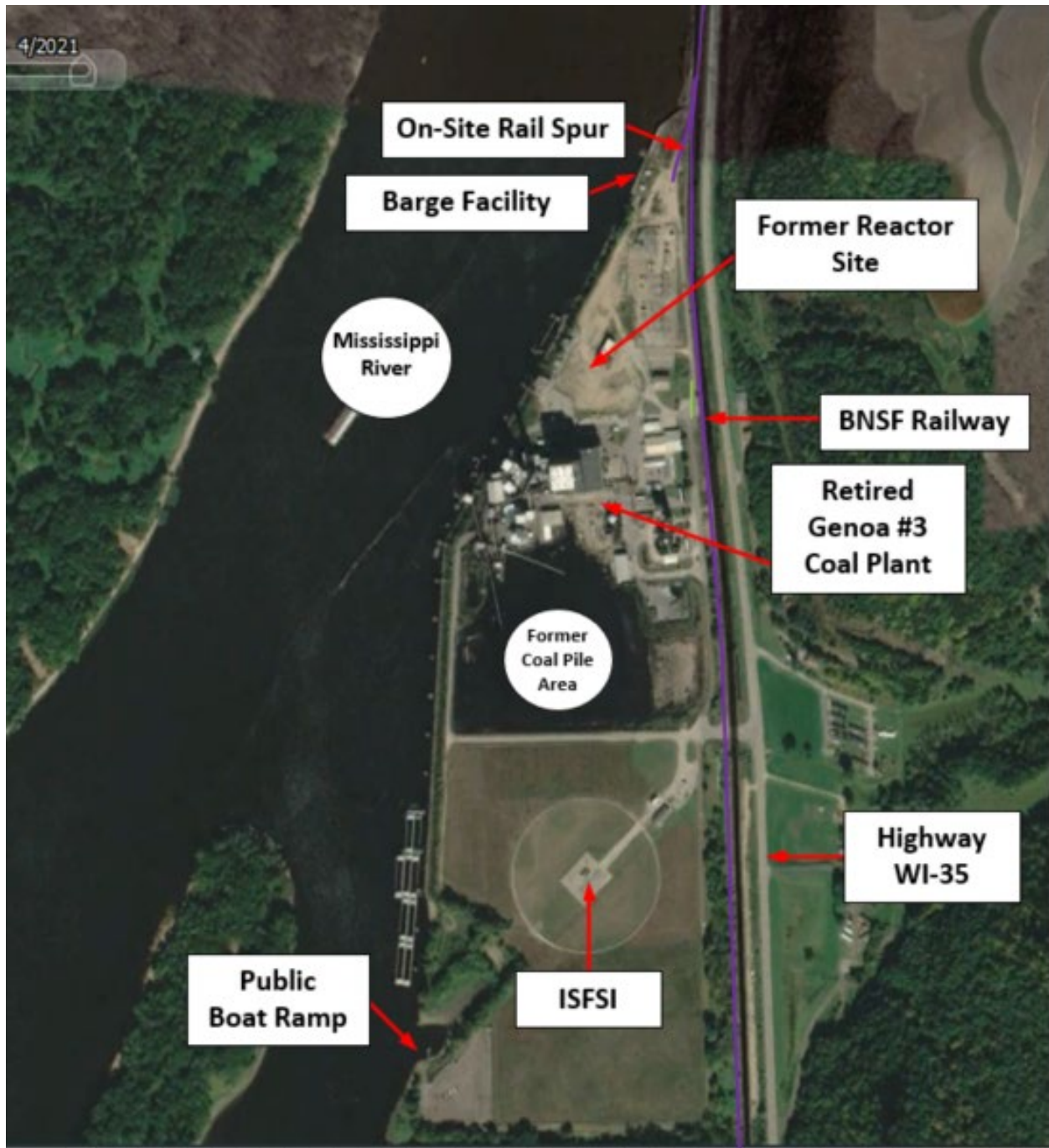
Figure 2-10: Aerial View of LACBWR Site [6]
