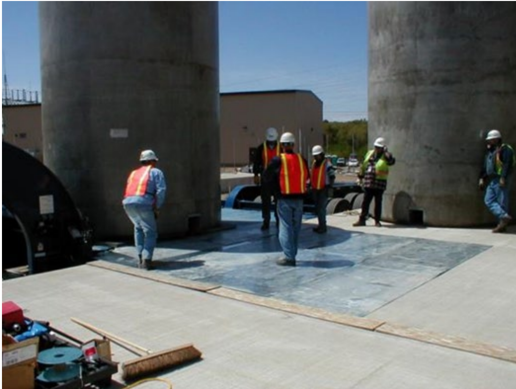
Figure 2-36: NAC VCC Movement From HHT to/from ISFSI Pad on Air Pads
