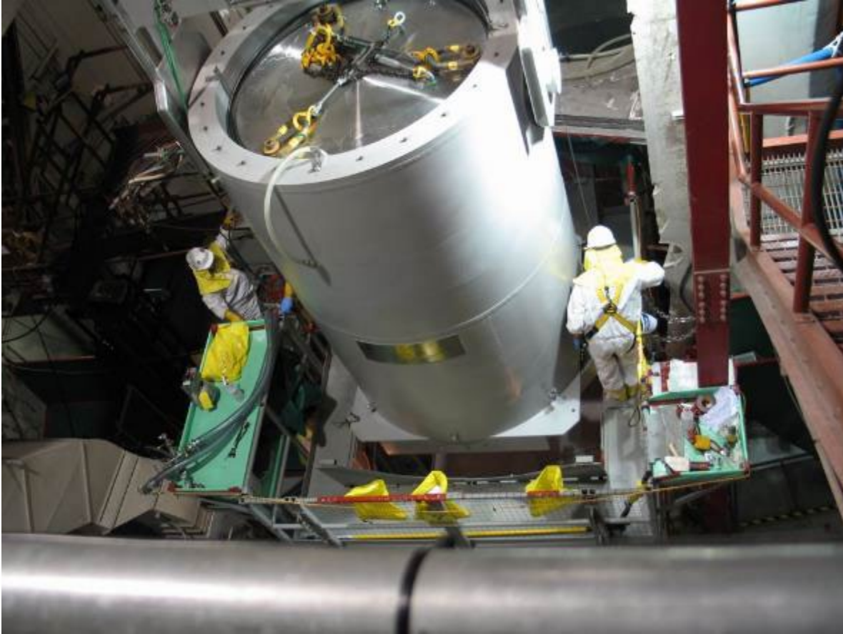
Figure 2-38: Loaded MPC-LACBWR TSC in TFR
