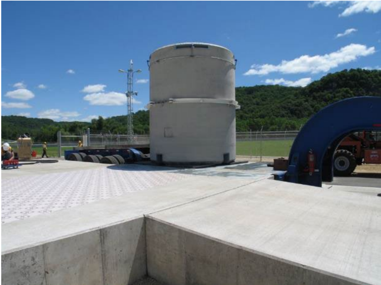
Figure 2-39: Loaded MPC-LACBWR VCC on HHT Ready for Movement to ISFSI Pad
