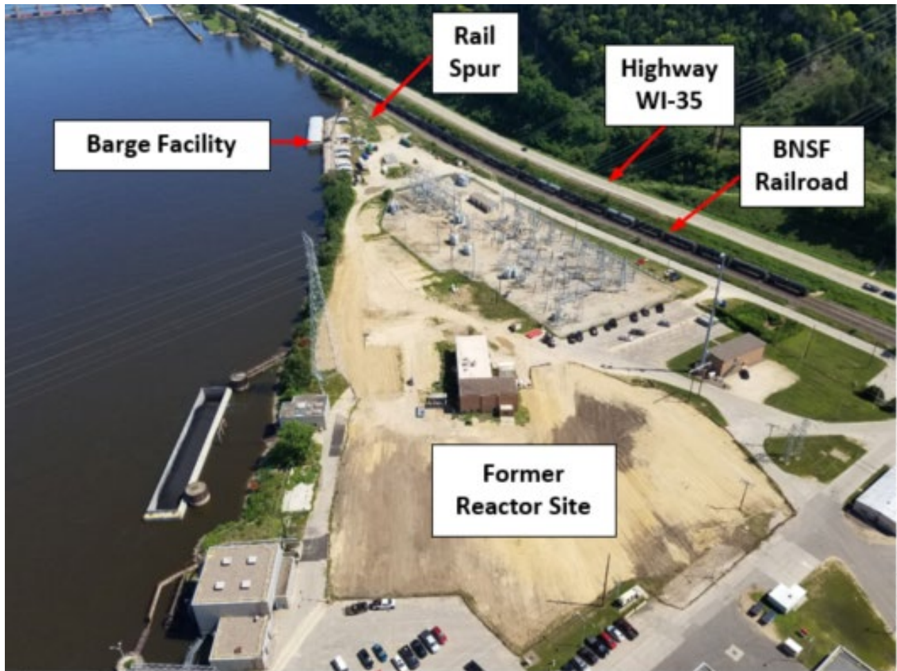
Figure 2-5: Former Reactor Site North View
