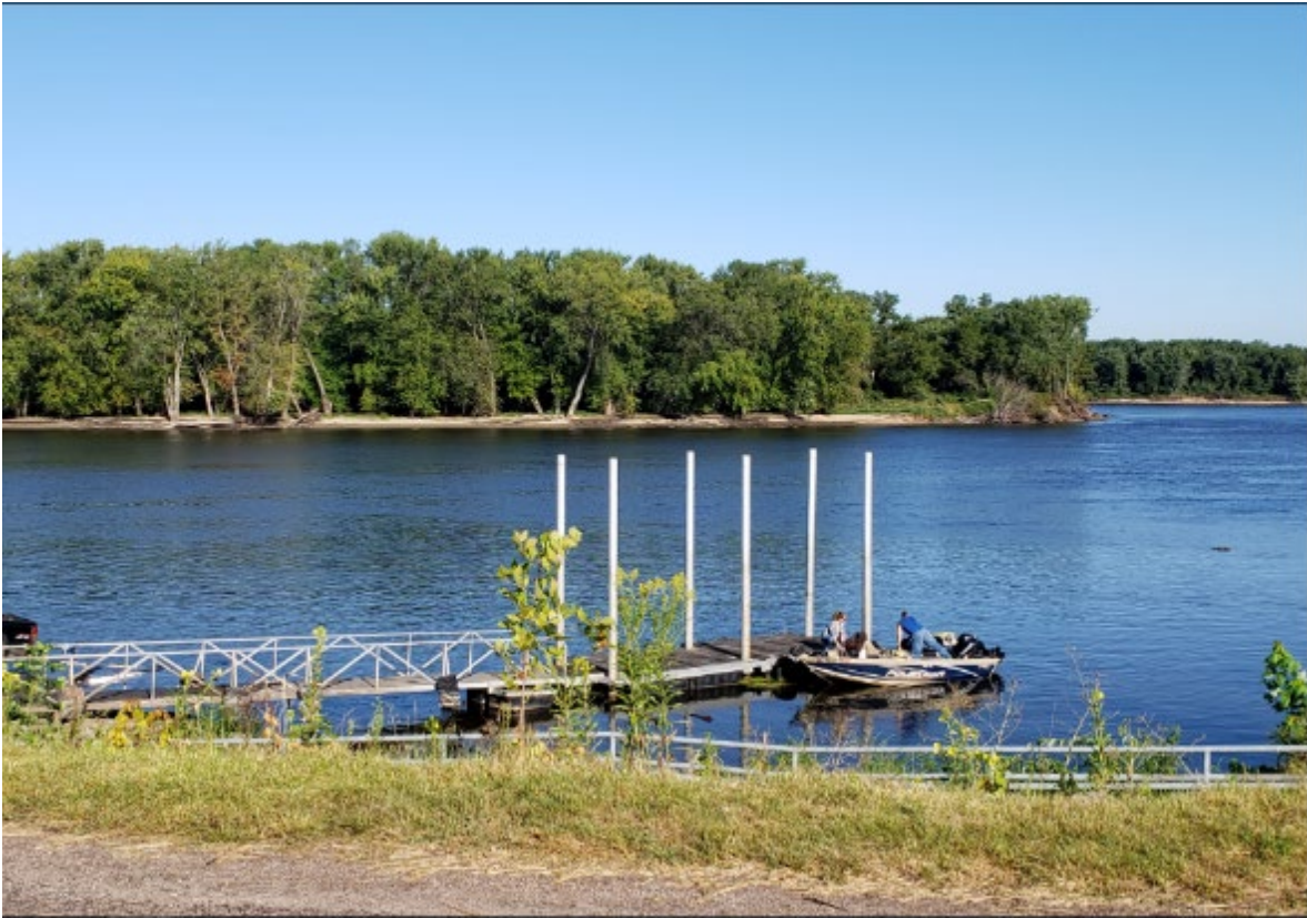
Figure 2-17: Pier at Boat Ramp Area
