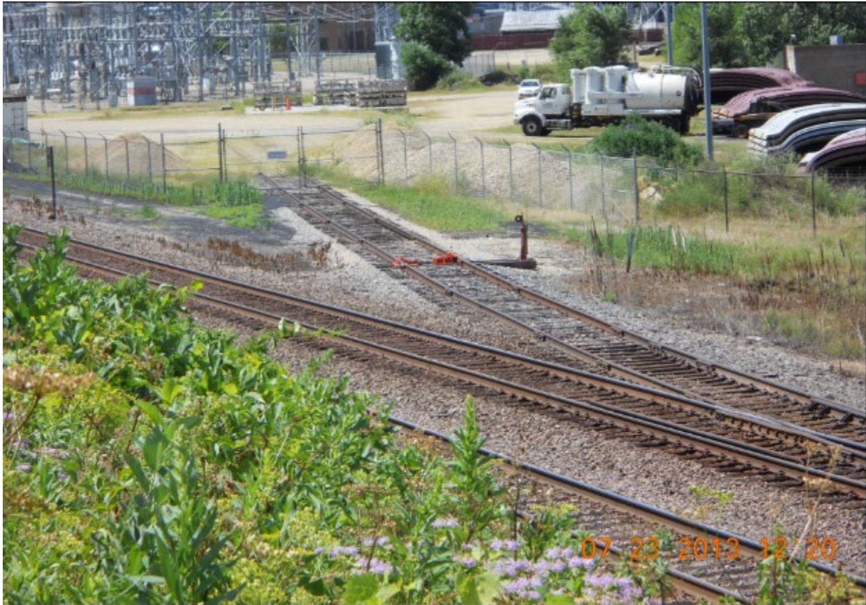
Figure 2-12: BNSF Main Line and On-Site Rail Spur
