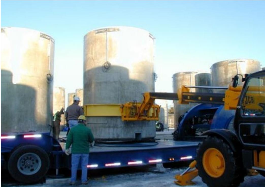
Figure 2-35: NAC VCC Movement from HHT to ISFSI Pad on Air Pads and Engaged to JCB Telescopic Handler
