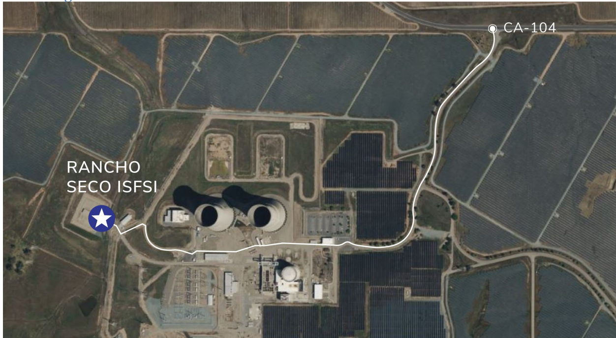
Figure 3-1: Path from the ISFSI Across the Site to the Nearest Public Road [1]
