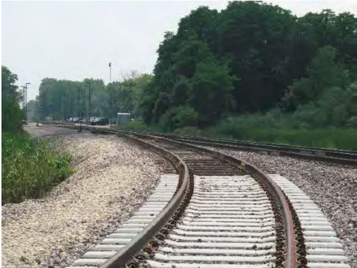
Figure 2-15: Junction of Zion On-Site Rail Spur with Union Pacific Railroad Showing Concrete Rail Ties (2013) 61
