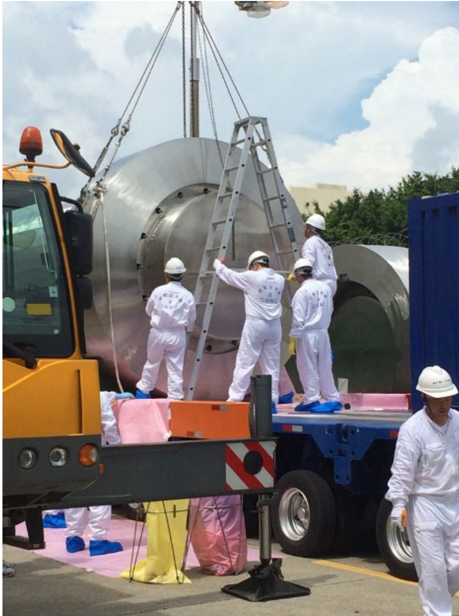
Figure 2-31: MAGNATRAN Package Impact Limiter Removal / Installation
