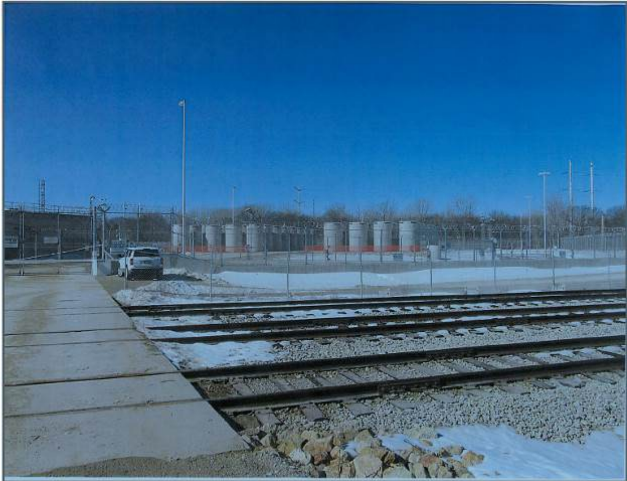
Figure 2-10: On-Site Rail Spur Adjacent to ISFSI [6]
