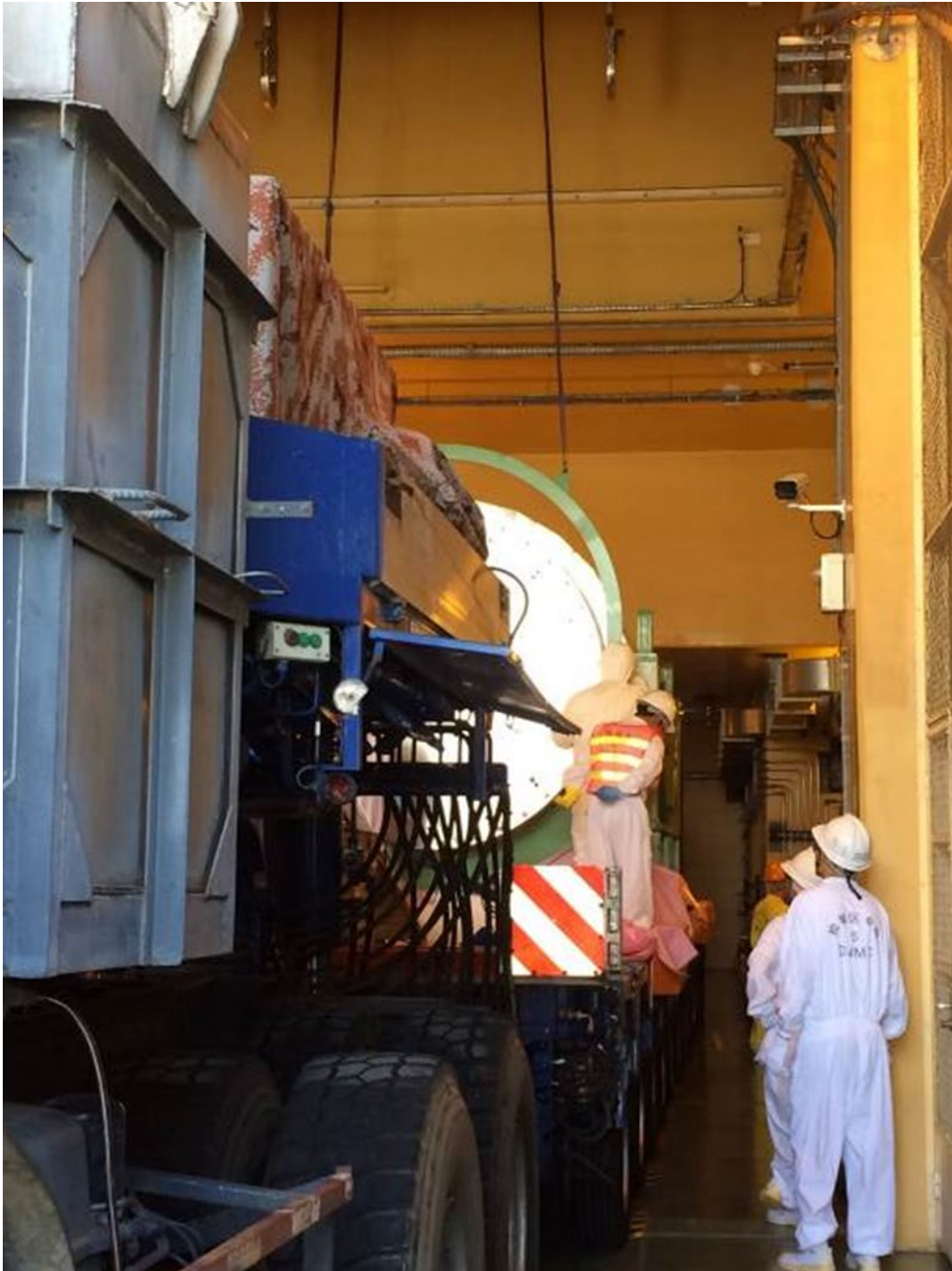
Figure 2-25: MAGNATRAN Package Front Tiedown Installation
