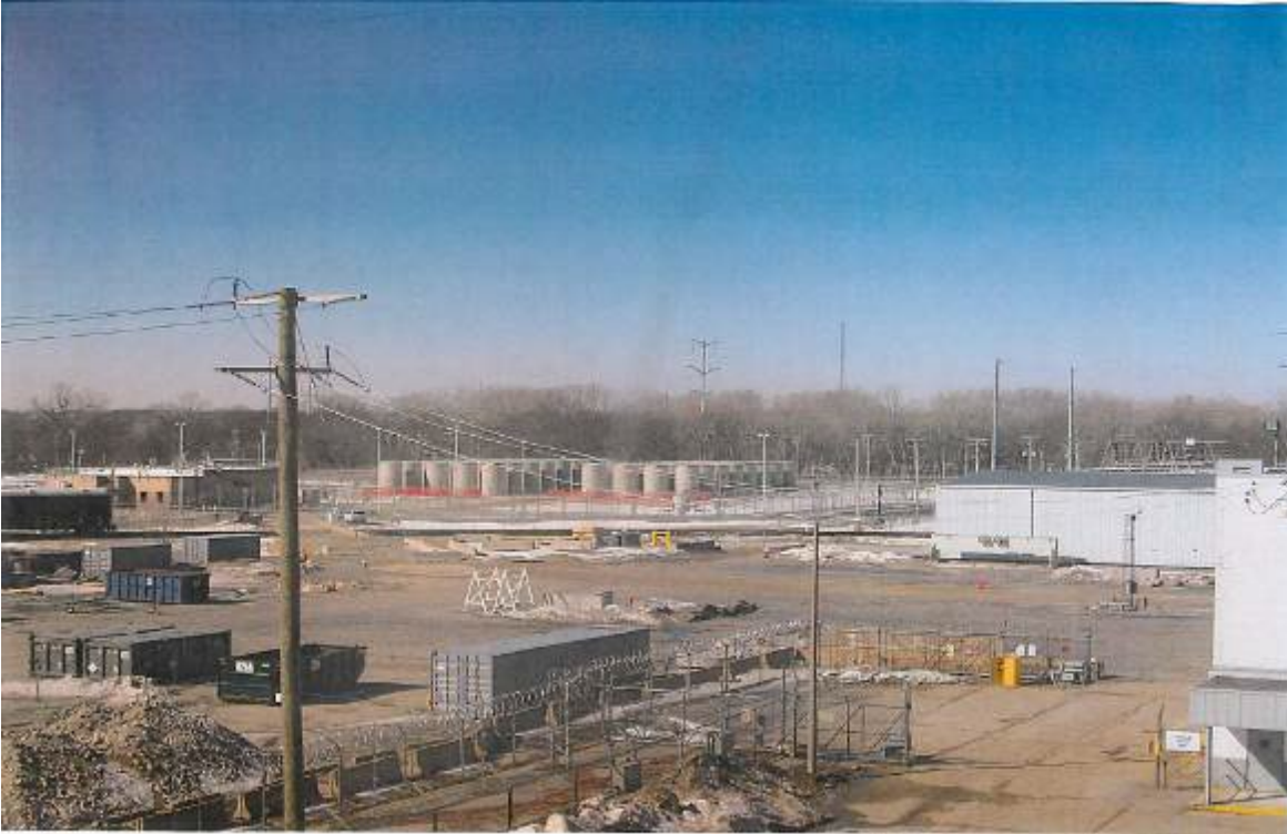
Figure 2-6: Zion ISFSI West View
