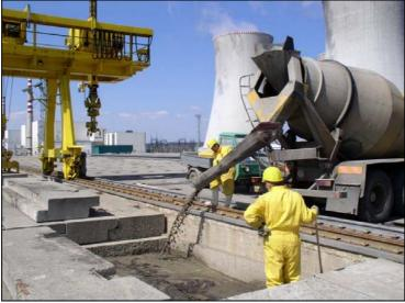
Fig. 8.3 Closing a full vault with concrete
