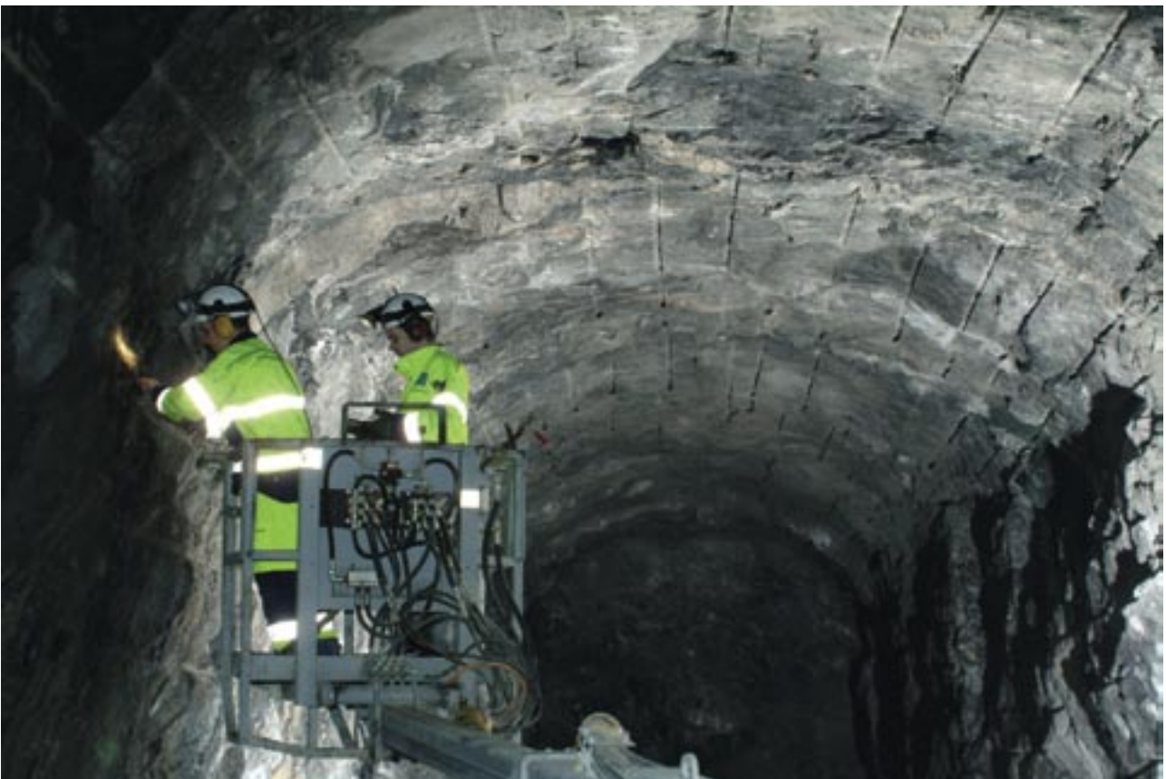
Figure 14. Geological mapping in the access tunnel of ONKALO.
