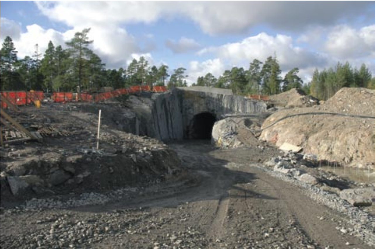
Figure 13. The opening of the ONKALO tunnel in October 2004.
