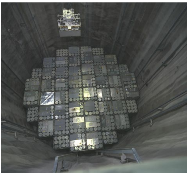
Figure 7. The Olkiluoto LILW repository. LLW drums in the disposal silo (left) and cross-sectional view of the repository lay-out (right).
