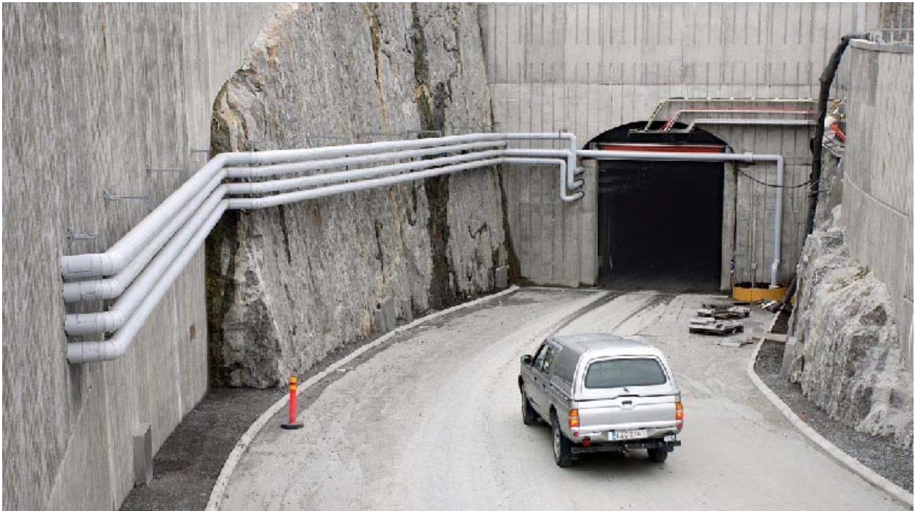
Figure 14. The opening of the ONKALO tunnel in 2007.
