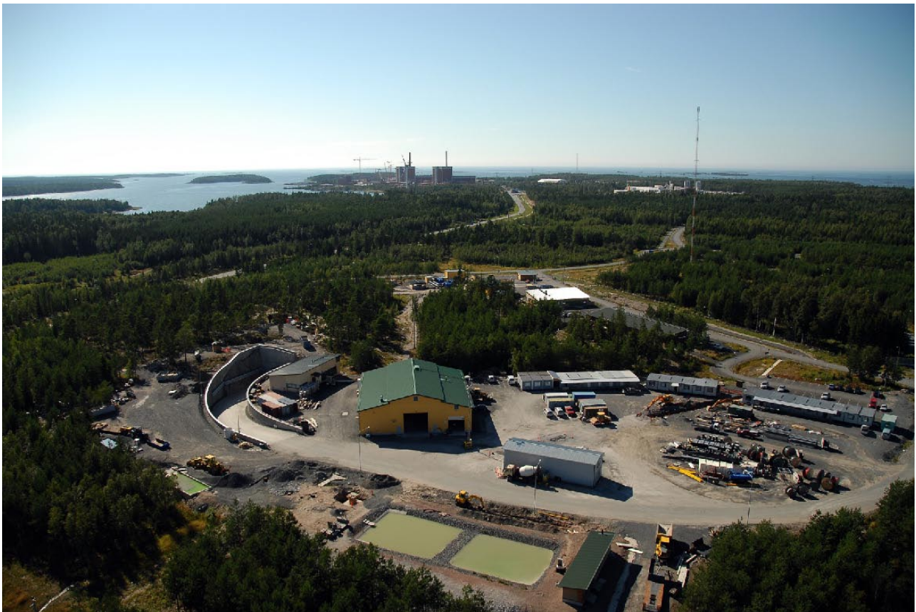
Figure 1. The access tunnel to the disposal facility of spent fuel under construction at Olkiluoto.
