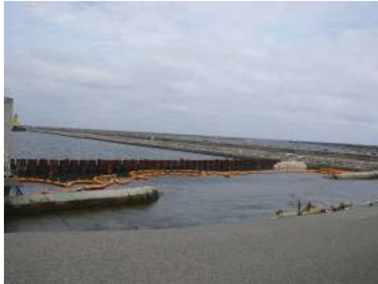
Status of steel pipe sheet pile
