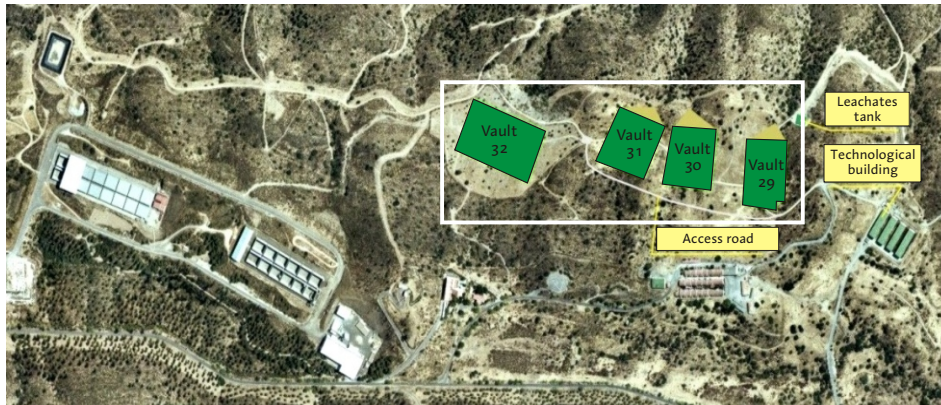
Figure 10. Aerial view of the very low level waste facility.
