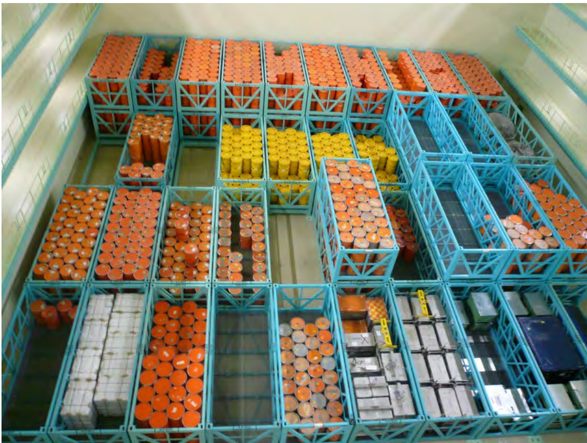
Figure 11: Storage hall for the storage of low level operational waste ZWIBEZ (Photo: ENSI)
