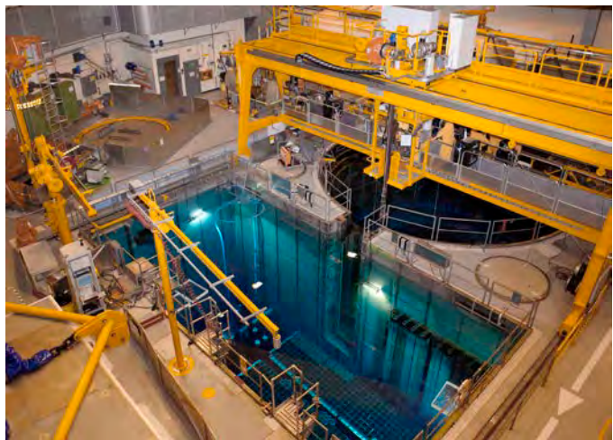
Figure 10: Spent fuel pond from the Mühleberg NPP (Photo: KKM)
