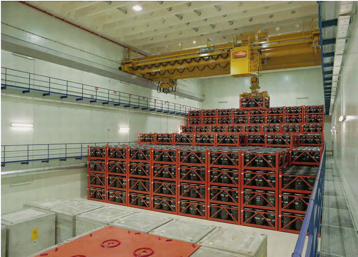
Figure 12: Storage hall for the storage of low level waste in the Federal Storage Facility (BZL) (Photo: PSI)
