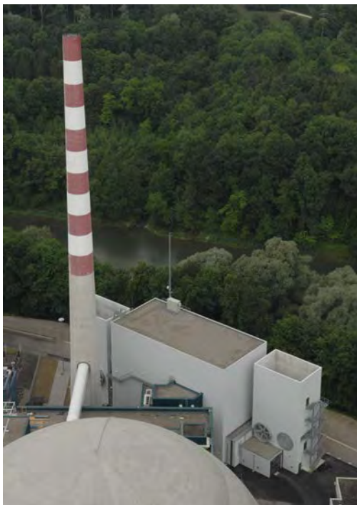
Figure 9: Gösgen NPP wet storage facility (Nasslager) (Photo: KKG)
