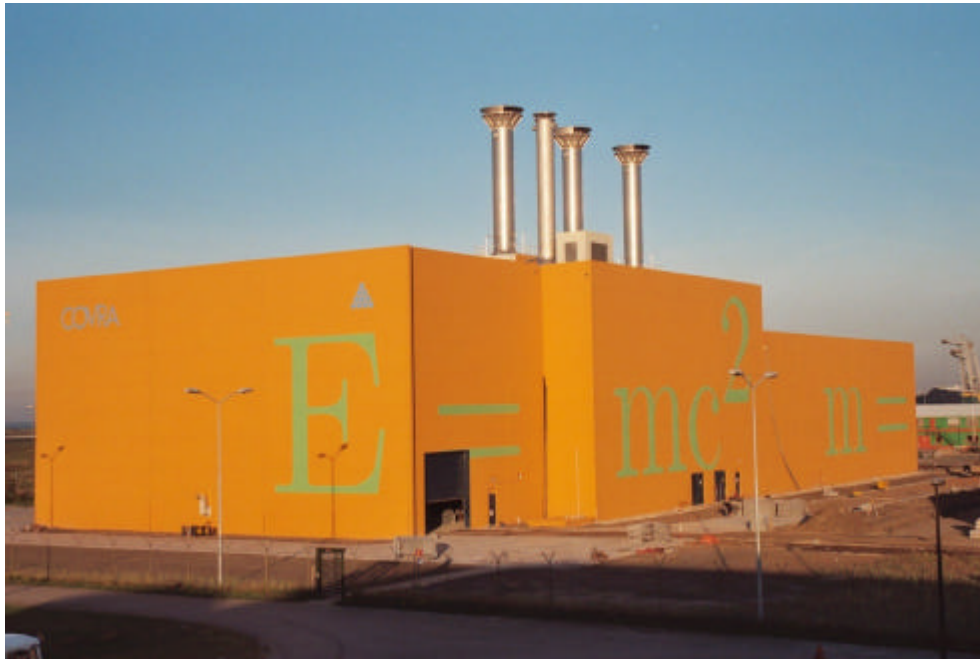
Figure 5. HABOG shortly before completion
